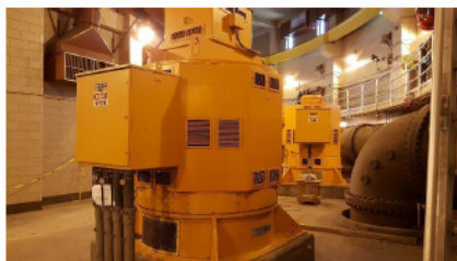
Main Raw Sewage Pumps at Pump Station 2
