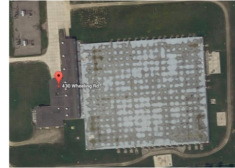
Imlay Pump Station
