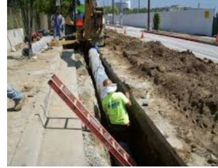
Water main being replaced
