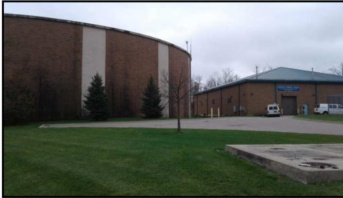
Figure VI-23. Haggerty Pump Station
