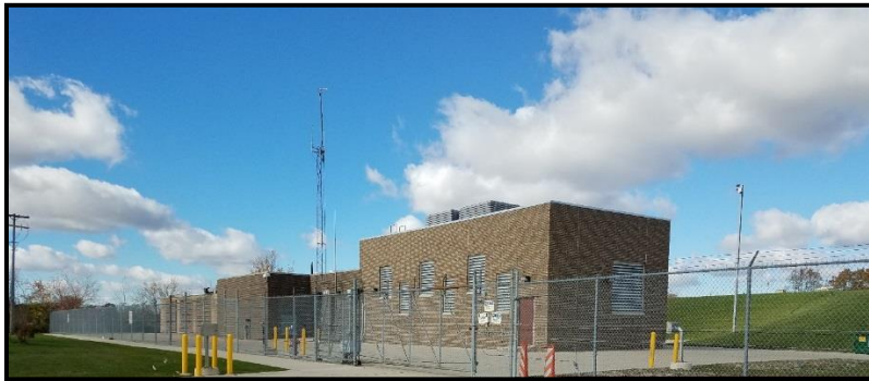
Figure VI-37. Wick Road Pump Station
