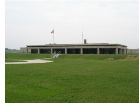
Lake Huron Water Treatment Plant
