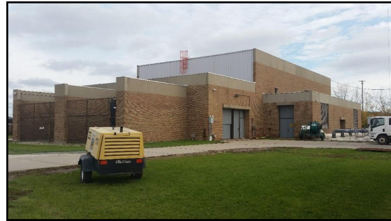
Figure VI-61. Northeast Pump Station
