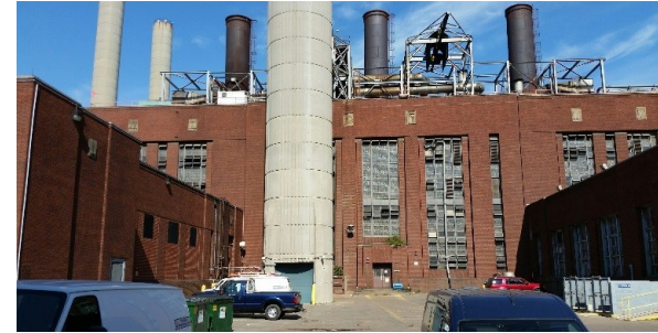
Complex – I Incinerator Building at the WRRF
