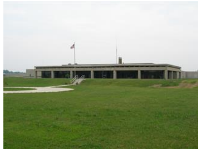
Figure VI-3. Lake Huron WTP
