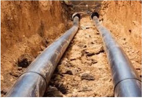
Example of pipe being laid
