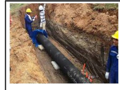
Water main being installed
