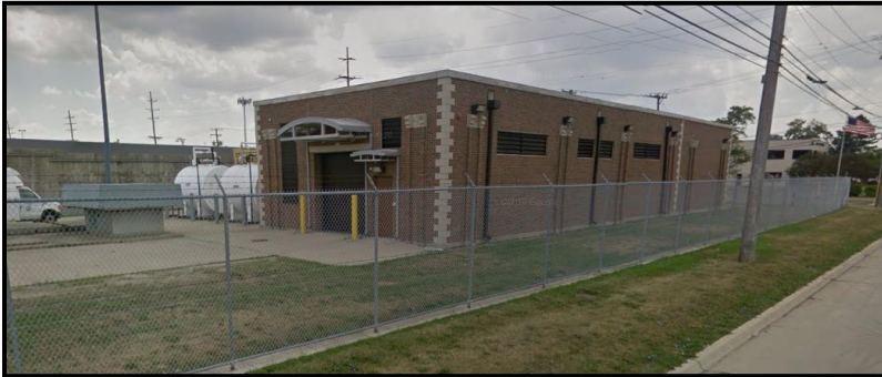
Figure VI-35. Schoolcraft Pump Station
