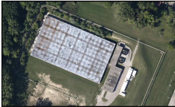
Figure VI-25. Franklin Pump Station
