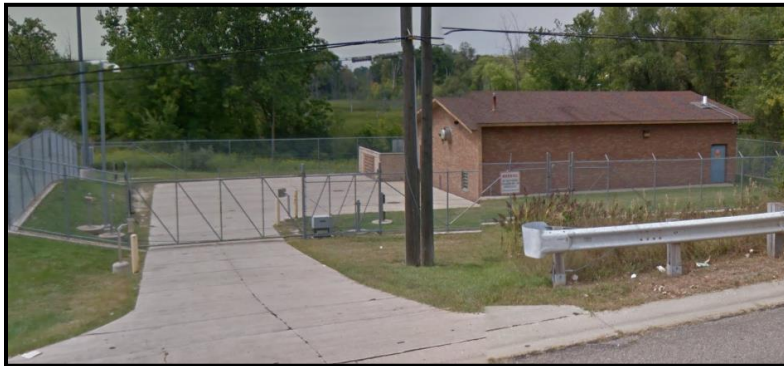
Figure VI-32. Orion Pump Station
