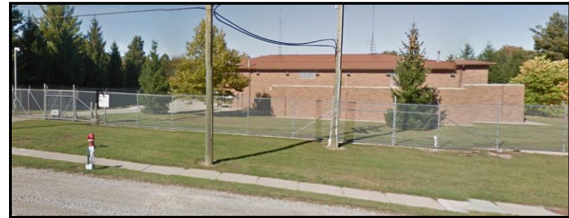
Figure VI-33. Rochester Pump Station
