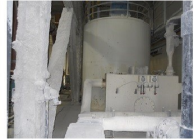
Powdered lime discharges into the COF causing lime to discharge throughout the building making the scrubber system to fail
