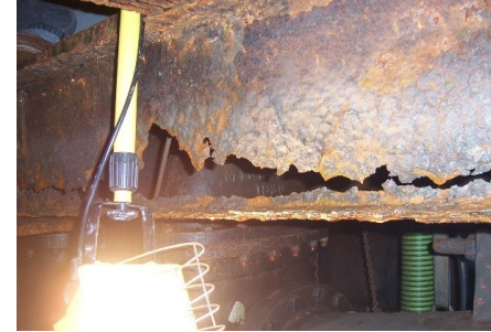
Deteriorated support beams holding up Low Lift Station. Dewatering and Sump Pumps at Elev. 42'-0" (left). Deteriorated grating and access ship's ladder in Low Lift Station - Looking down at Elev. 50'-0" and 42'-0" from Elev. 62'-0" (right).
