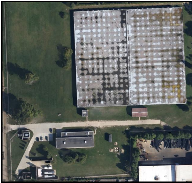
Figure VI-34. West Service Center
