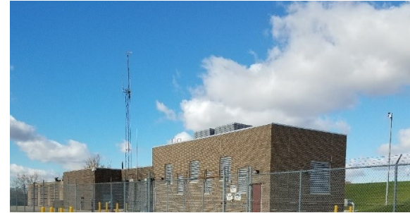
Wick Road Station
