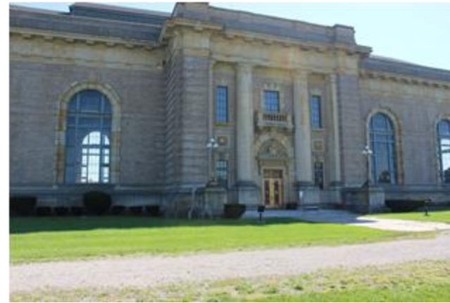
Figure VI-10. Water Works Park WTP
