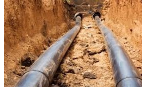
Water main installation
