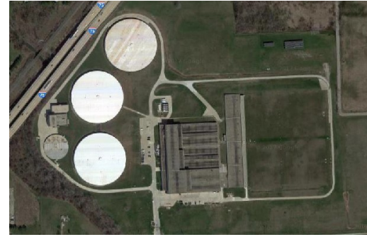
Aerial view of the Southwest Water Treatment Plant
