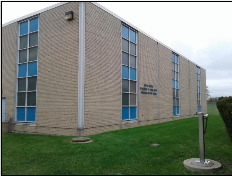
Figure VI-29. Newburgh Pump Station
