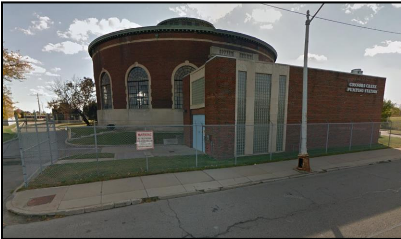
Figure VI-55. Conner Creek Pump Station
