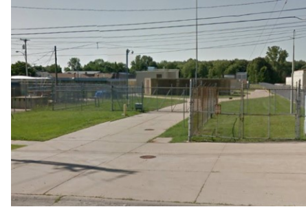
Joy Road Pumping Station
