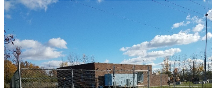
Ypsilanti Pump Station
