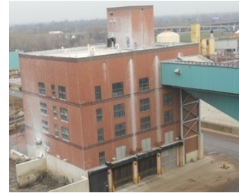
Powdered lime discharges into the COF causing lime to discharge throughout the building making the scrubber system to fail
