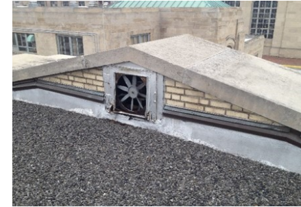
Springwells filter building
