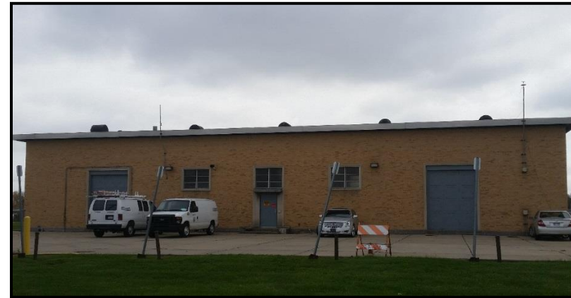
Figure VI-30. Northwest Pump Station
