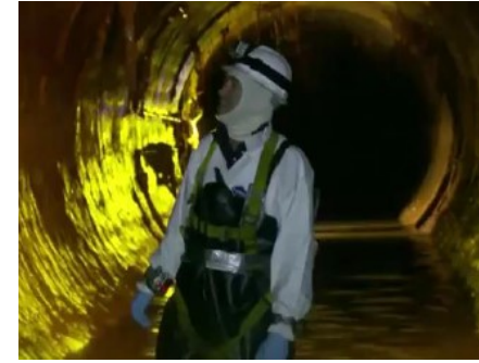
Example inspection of a large sewer
