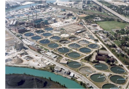
Aerial view of the WRRF
