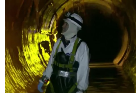
Visual inspection of a large sewer
