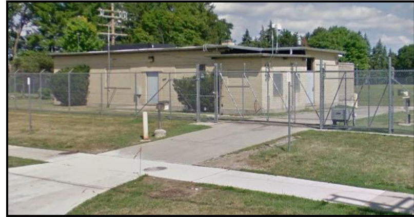
Figure VI-36. West Chicago Pump Station
