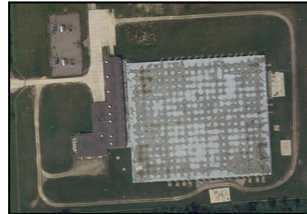
Figure VI-28. Imlay Pump Station
