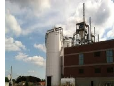
New GLWA Biosolids Dryer Facility
