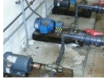
Retrofitted chemical feed pump replacement at Puritan-Fenkell RTB and makeshift wooden stairs to enter Basin Valve Gallery
