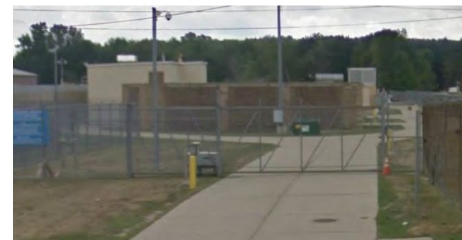
Figure 27. Joy Road Pump Station
