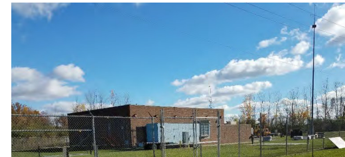
Figure 38. Ypsilanti Pump Station
