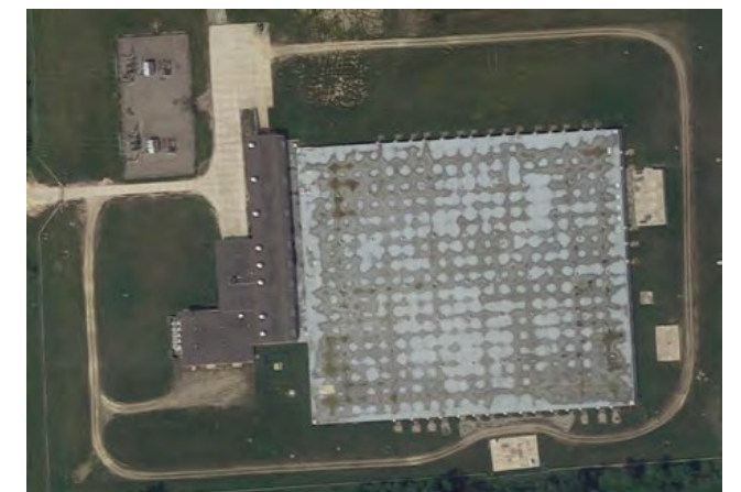
Figure 28. Imlay Pump Station
