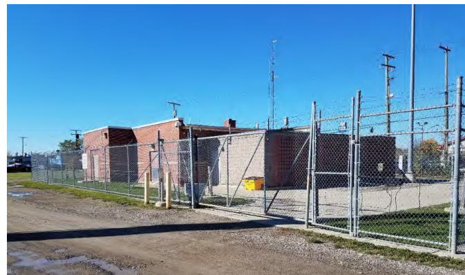
Figure 26: Michigan Avenue Pump Station
