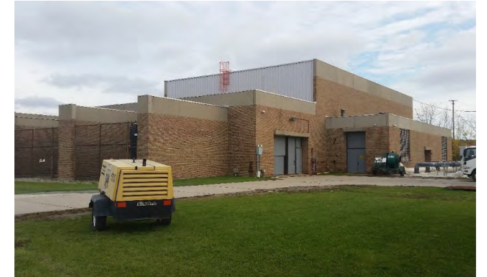
Figure 61. Northeast Pump Station
