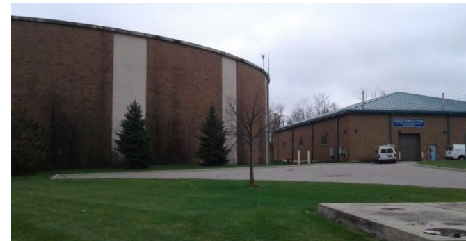
Figure 23: Haggerty Pump Station
