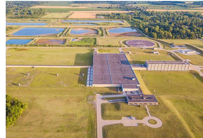
Figure 3. Lake Huron WTP
