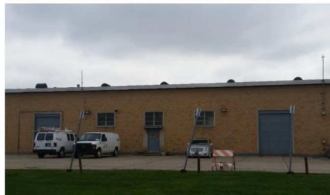
Figure 30: Northwest Pump Station
