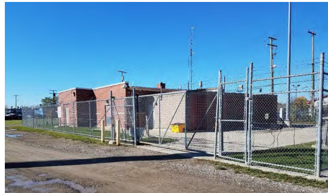
Figure 26: Michigan Avenue Pump Station
