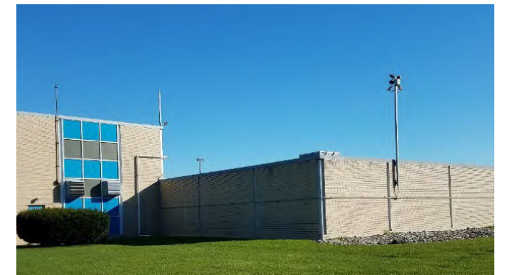
Figure 24: Ford Road Pump Station
