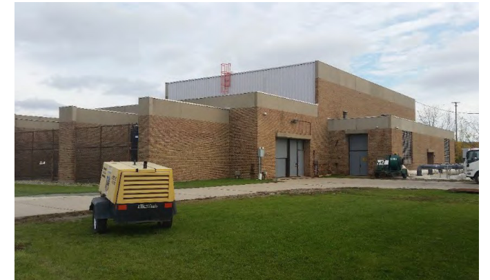
Figure 61. Northeast Pump Station
