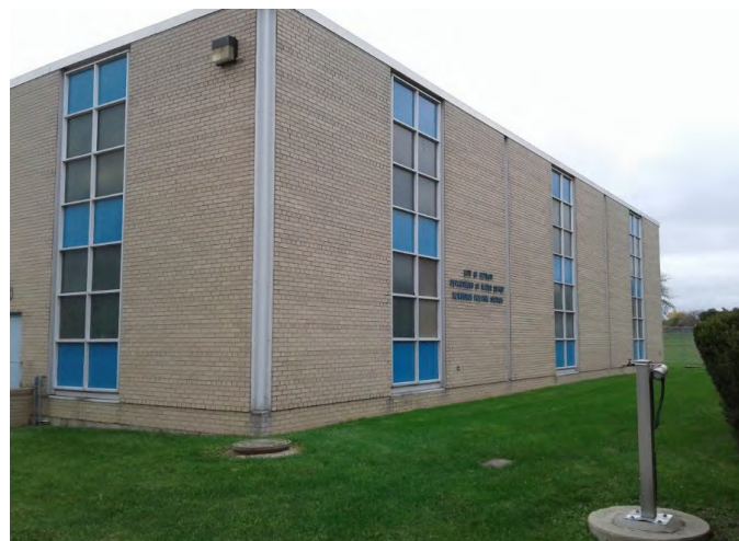
Figure 29. Newburgh Pump Station
