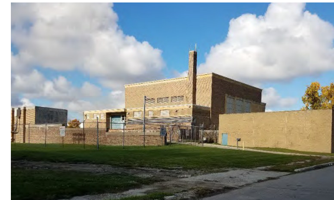
Figure 59. Freud Pump Station
