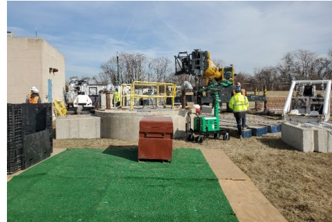
Mobilization at existing access shaft
