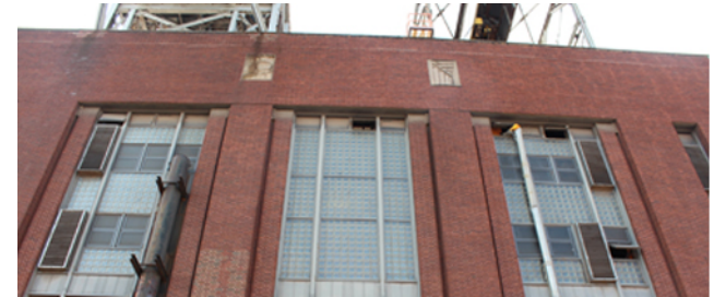
WRRF Roof Replacement for Multiple Facilities Program
