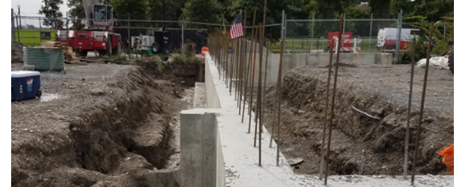
Fairview Pumping Station - Replace Four Sanitary Pumps
