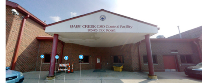
Baby Creek CSO Facility Influent Flushing System
