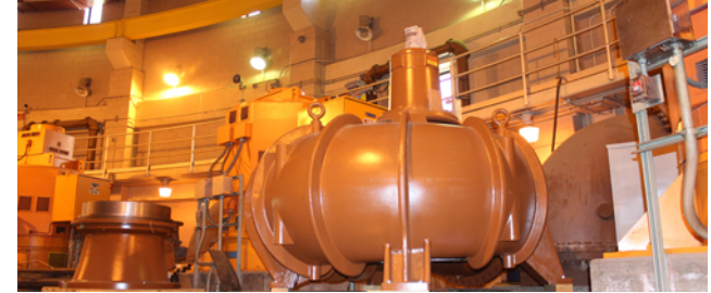
WRRF PS No. 2 Improvements Phase II
