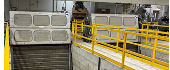
CSO Baby Creek Screen Rehabilitation
