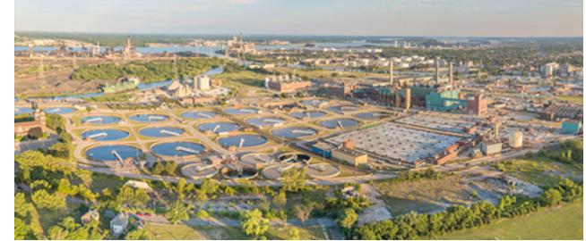
WRRF Rehabilitation of the Secondary Clarifiers Phase 1
