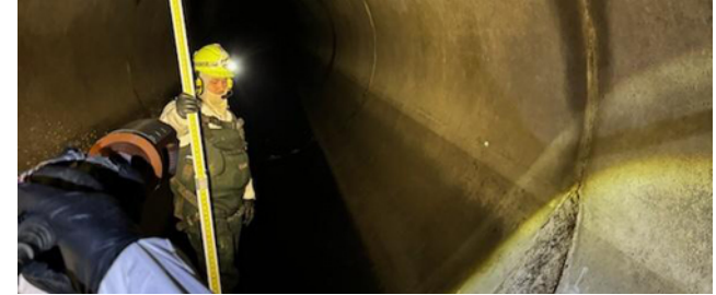
Emergency and Urgent Sewer Repair II
