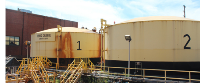
WRRF Rehabilitation of Ferric Chloride Feed System in PS-1 and Complex B Sludge Lines
