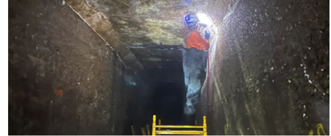
Conveyance System Repairs (Outfalls)
