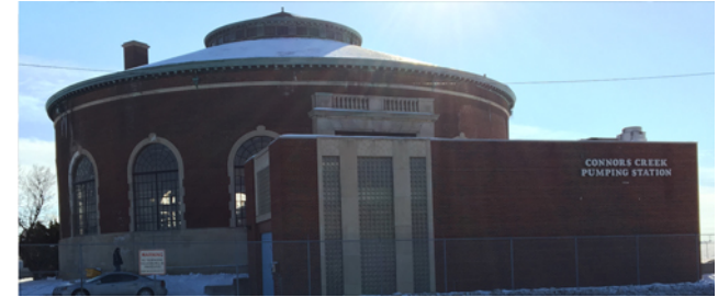
Conner Creek Pump Station Improvements
