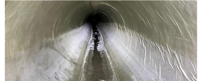
Sewer Rehabilitation and Repair
