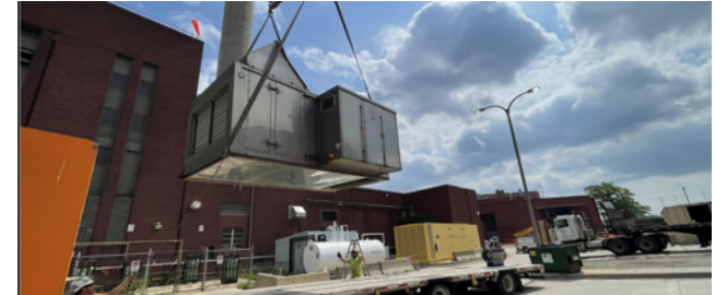
PS 1 Rack and Grit HVAC System Upgrade
