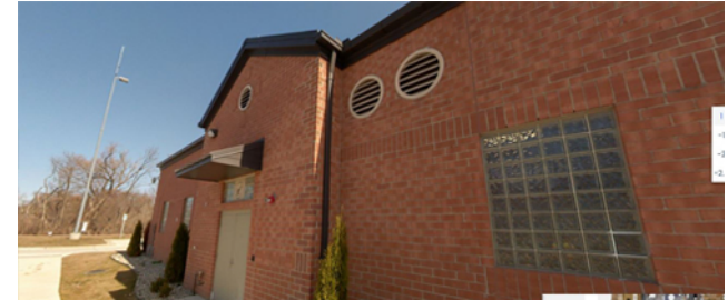
HVAC Improvements at Puritan Fenkell and Seven Mile CSO Facilities
