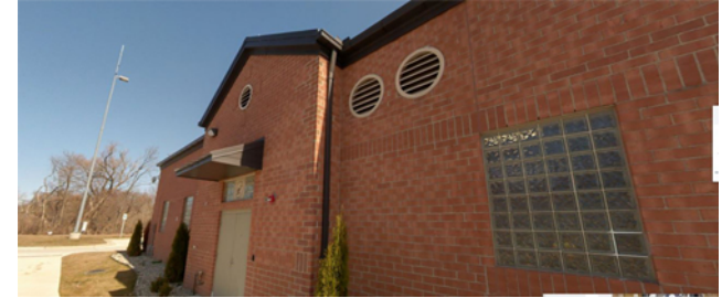
Conversion to Complete Capture Basin at Puritan Fenkell and Seven Mile CSO Facilities
