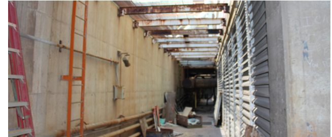
WRRF Structural Improvements
