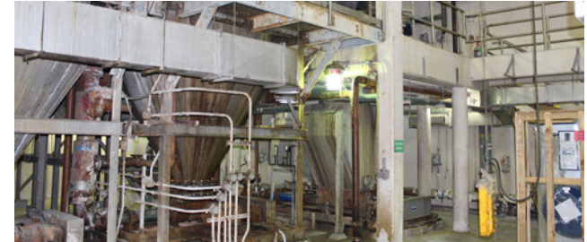
WRRF Rehabilitation of the Circular Primary Clarifier Scum Removal System
