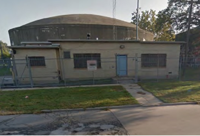
Figure 22. Electric Avenue Pump Station
