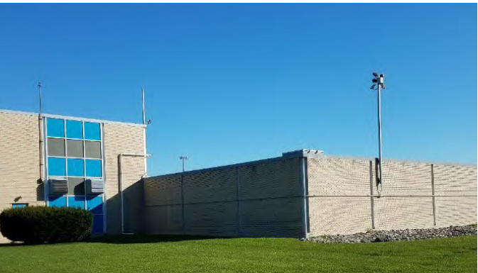
Figure 24: Ford Road Pump Station
