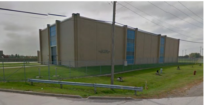
Figure 31. North Service Center
