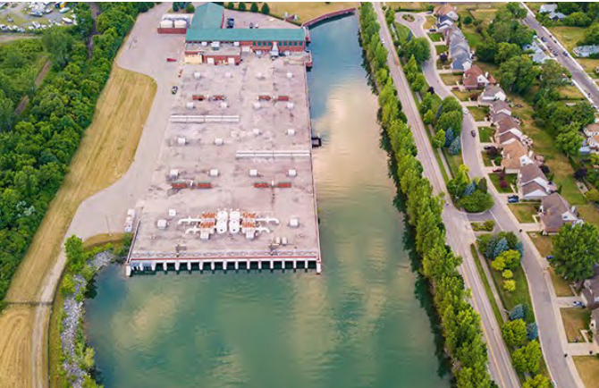
Figure 40. Conner Creek CSO RTB
