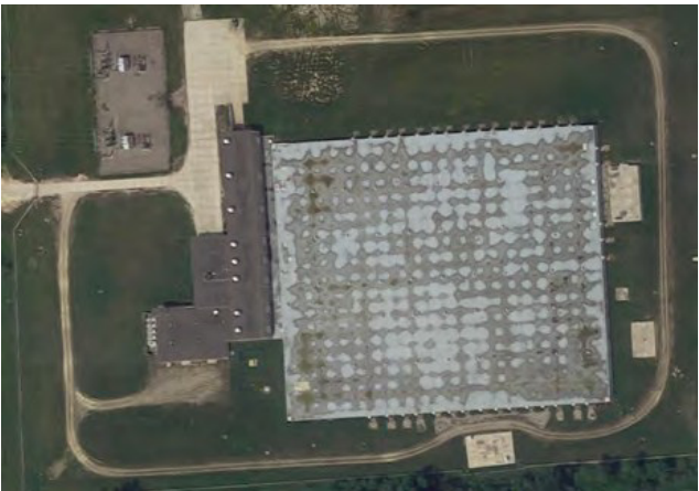
Figure 28. Imlay Pump Station
