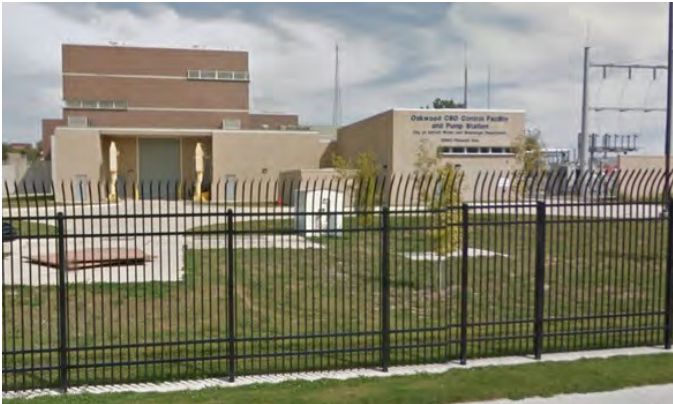
Figure 62. Oakwood Pump Station
