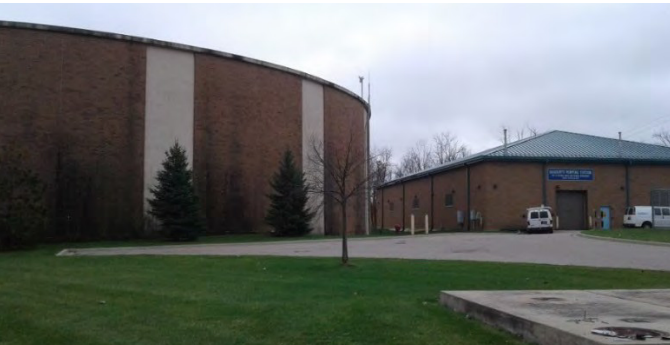
Figure 23: Haggerty Pump Station
