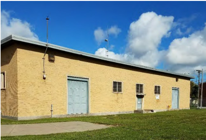
Figure 21. Eastside Pump Station
