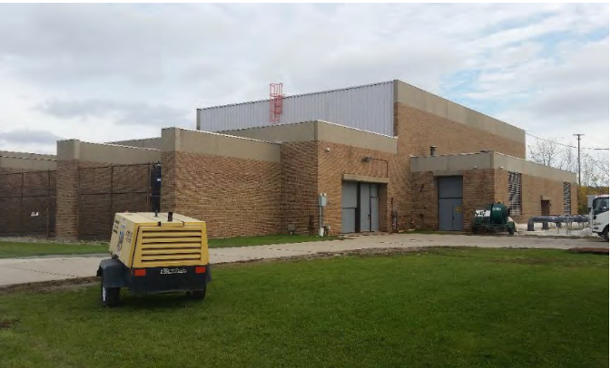
Figure 61. Northeast Pump Station
