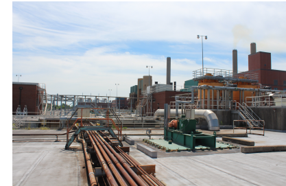
Aeration Basin 1 and ILP's 1 and 2
