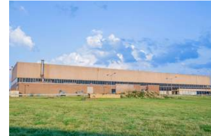
SW SCADA System Upgrade
