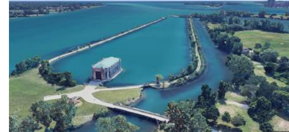
Aerial image of Belle Isle intake structure and lagoon.
