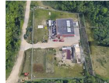
Existing Ypsi station
