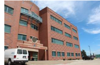
New Administration Building
