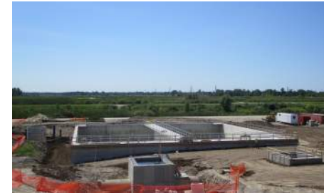
Overall progress photo that shows new WWRB, JS1, JS2 and SPS 8/20/20
