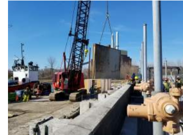
Effluent Relief Gate Repair
