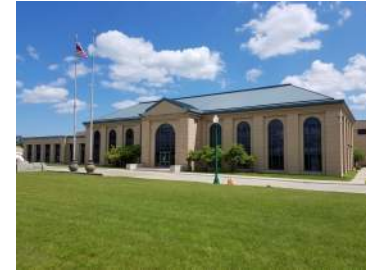
Water Works Park Water Treatment Plant
