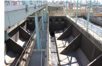
Pump Station 2, Grit channels
