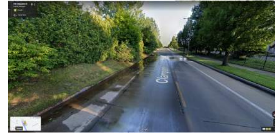
Photo of the berm leaking into Clairpointe
