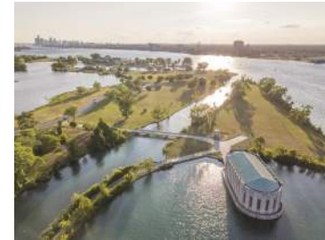
Belle Isle Intake
