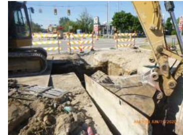
Construction on Merriman Rd.
