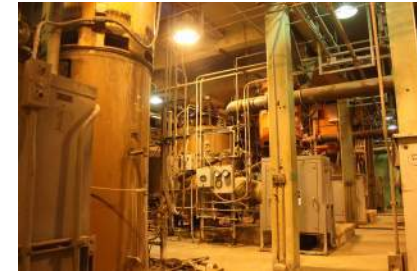
SFE Building, Basement
