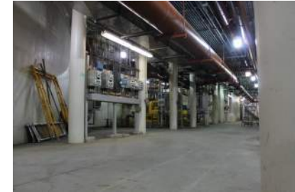
Complex B, Basement
