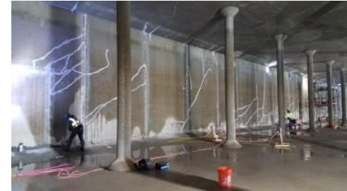
Imlay Booster Station: Sealing interior wall cracks
