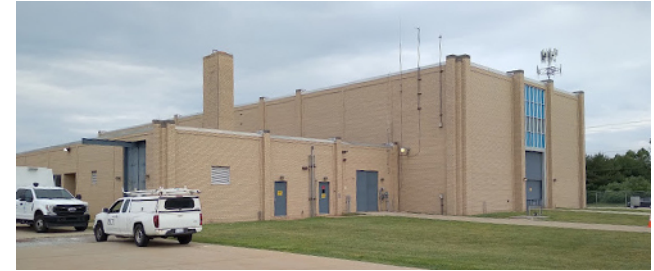
North Service Center Pumping Station
