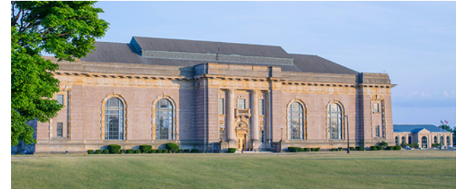
Water Works Park
