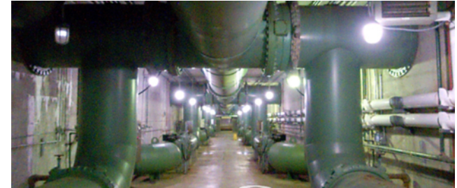
WTP Filtration Improvement
