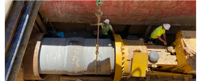
Wick Road Water Transmission Main
