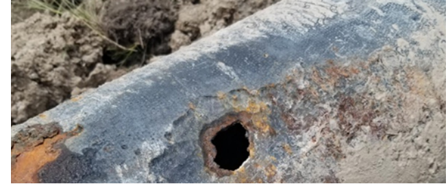
Fireloop and Plant Water Improvements
