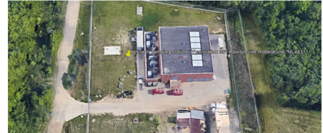
Ypsilanti Booster Pumping Station
