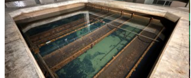
Northeast Water Treatment Plant Filter Replacement
