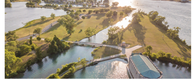
Belle Isle Intake System
