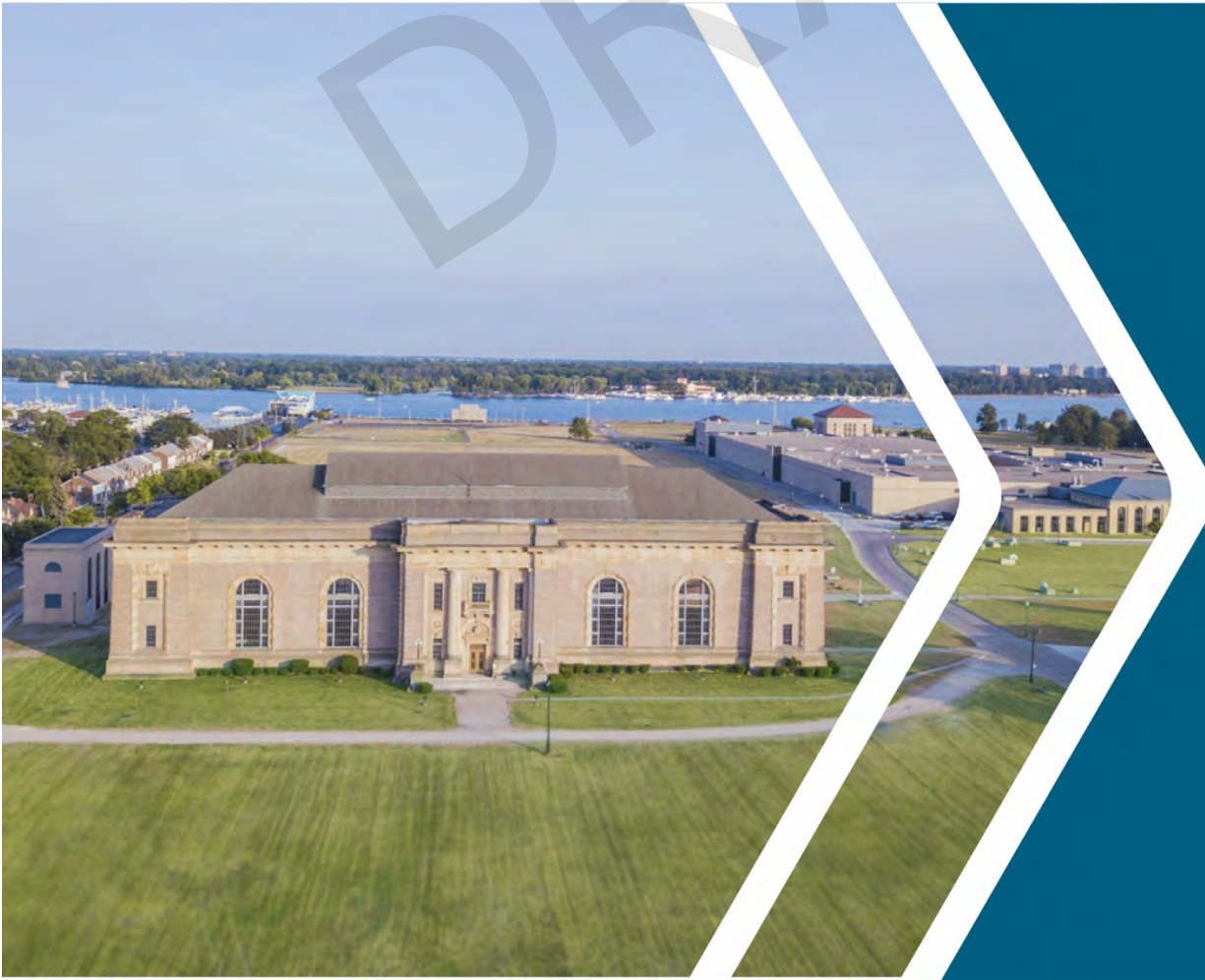
Water Works Park Water Treatment Facility
