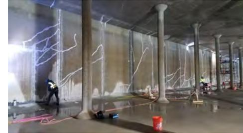
Imlay Booster Station: Sealing interior wall cracks
