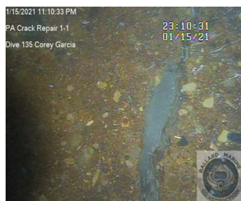
Pennsylvania Crack Repair-After Injection
