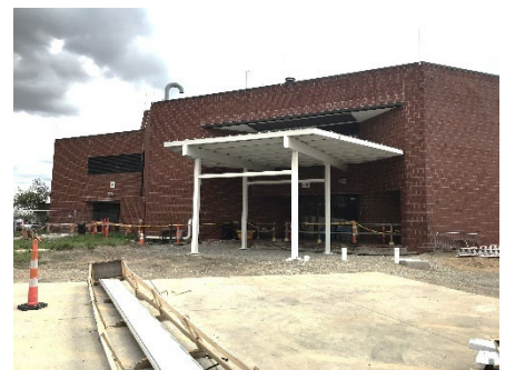
Ragland Canopy Installed
