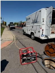
Water pump used to drain manhole
