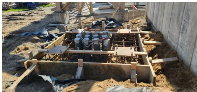
Foundation structural support for conduct
