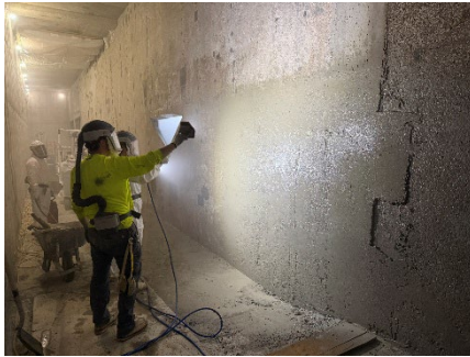
Waterproofing the flow channel walls
