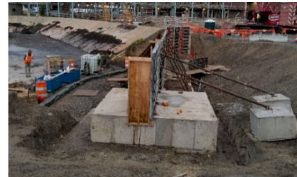
Ash Lagoon Concrete Work Progress
