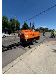
Air compressor for powering jack
