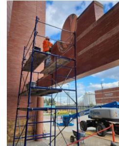
Caulking replacement at NAB
