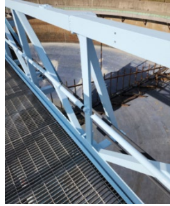
New paint on railing at Tank #1
