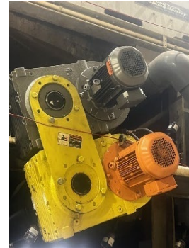
New upper belt installed on BFP
