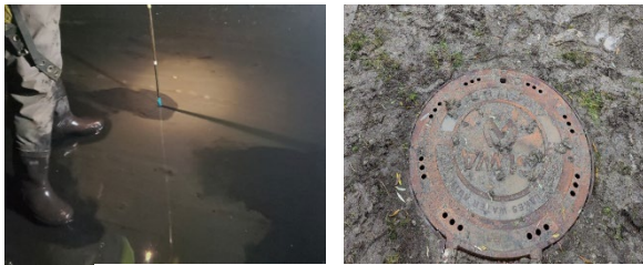
Cleaned West Barrel New GLWA Manhole
