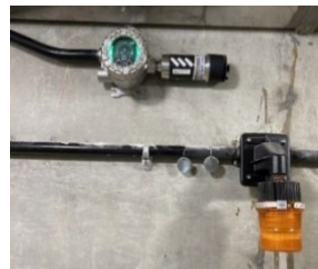
E/M Building Gas Sensor
