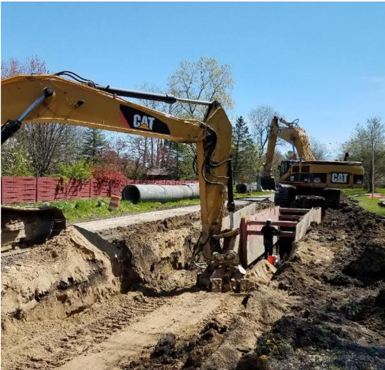
*Positioning of Transition Pipe Prior to Placing Lid on Vault Structure*
