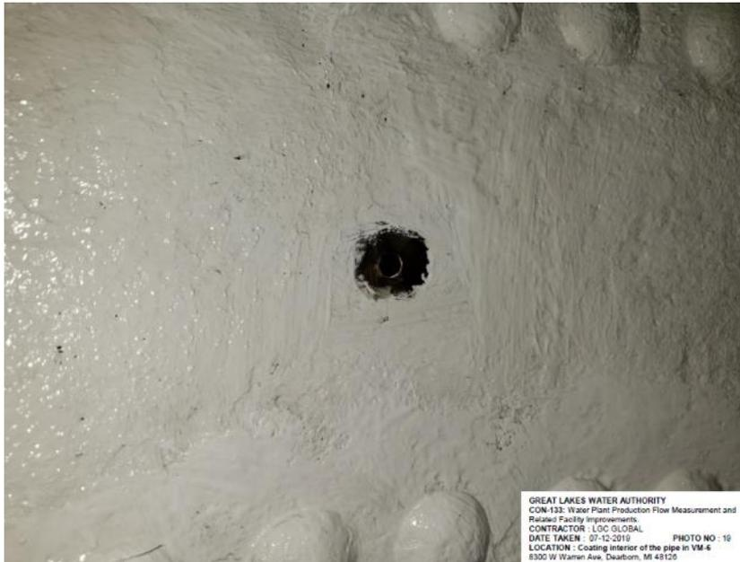
*Rehabbed pressure port for venturi meter*
