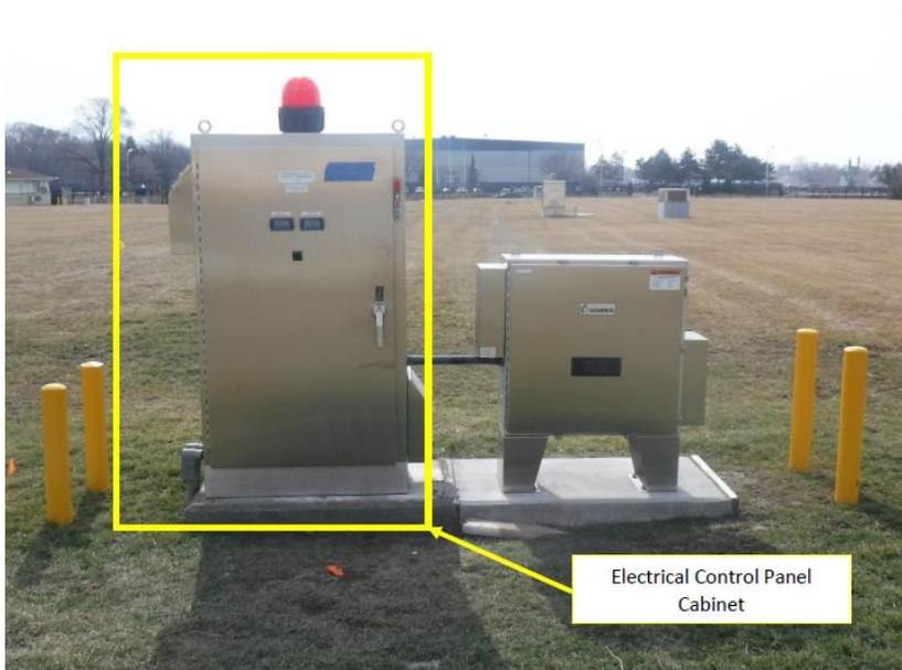
*Typical new VM-6 Flood float/switch and sum pumps system.*
