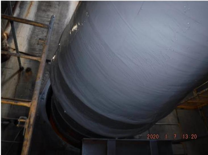
*VM-5 Exterior after coating with Belzona 5812 DW coat*
