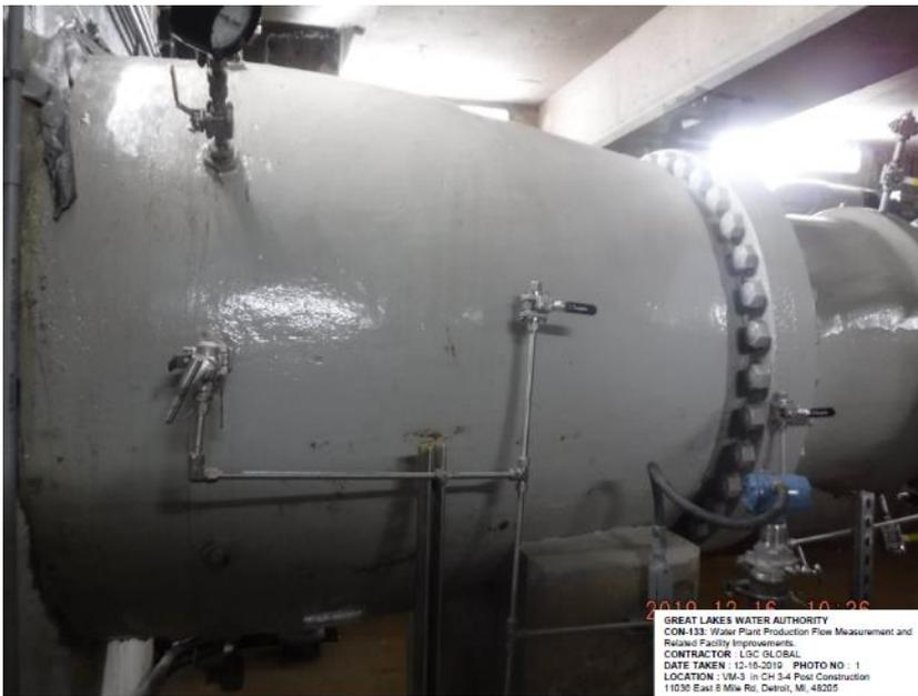
*Venturi meter exterior no. 3 before rehab*
