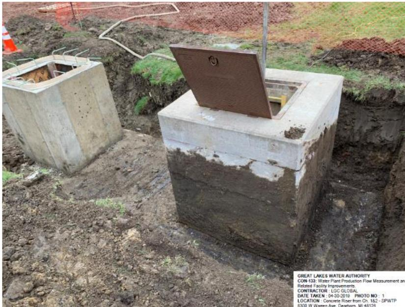
*Water proofing concrete risers for metering chamber*
