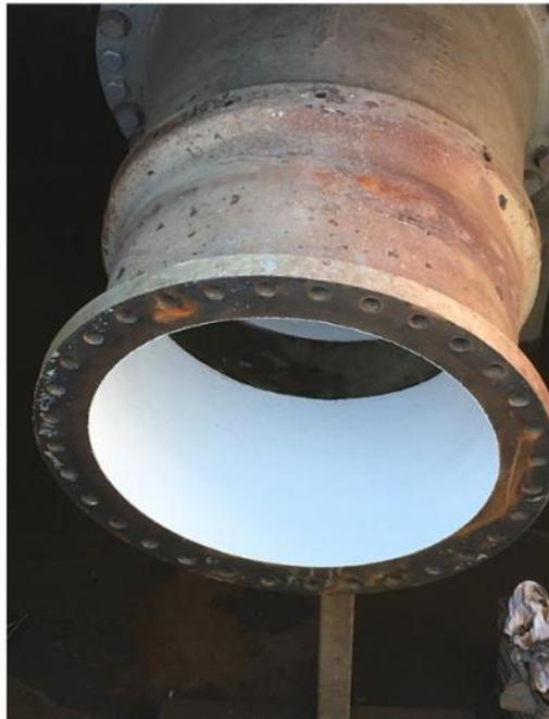
*Photo 3: Second coat of paint applied at the divergent section of VM-6 at the NEWTP.*
