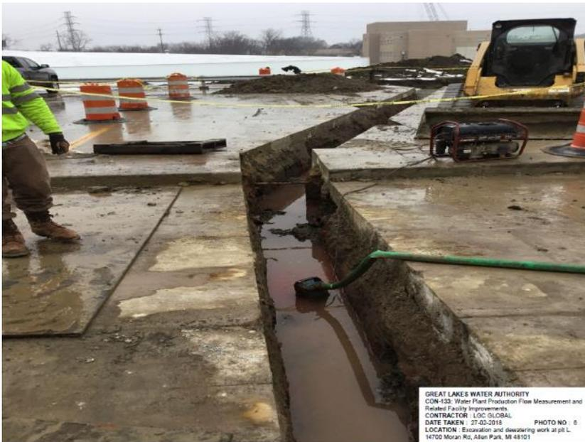
*Removing concrete riser at chamber L*
