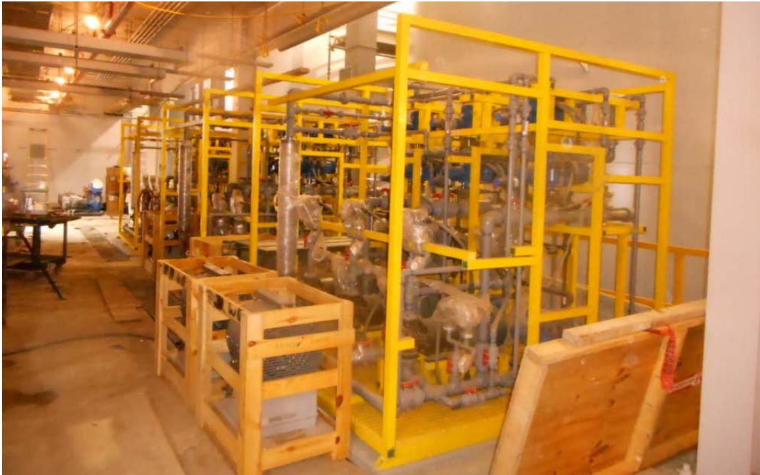
Installation of chemical metering pumps is in progress
