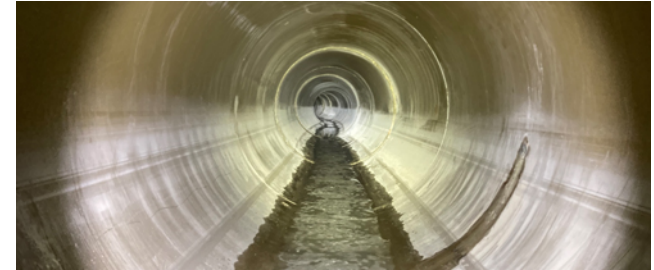
B-39 Outfall Rehabilitation
