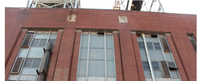
WRRF Roof Replacement for Multiple Facilities Program
