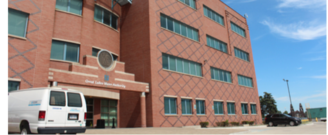
WRRF 4th Floor Renovation
