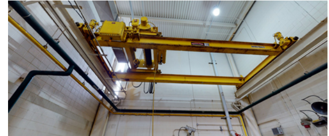
Oakwood HVAC Project
