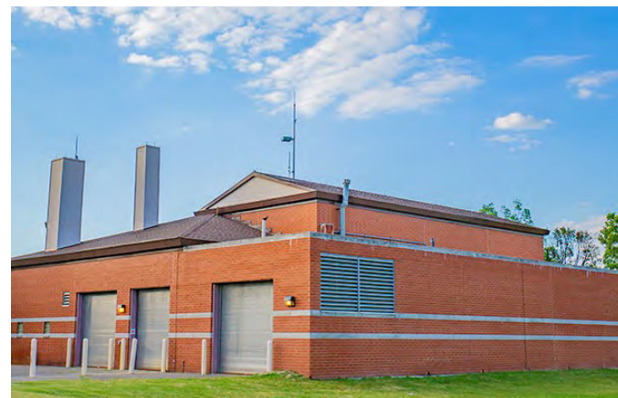
Figure 43. Puritan-Fenkell CSO RTB
