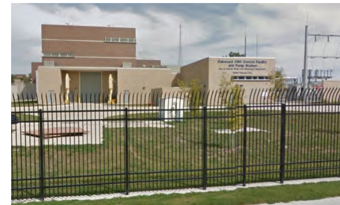
Figure 62. Oakwood Pump Station
