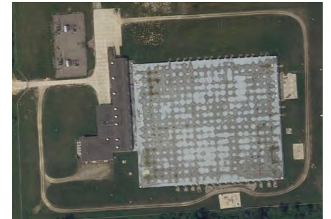
Figure 28. Imlay Pump Station
