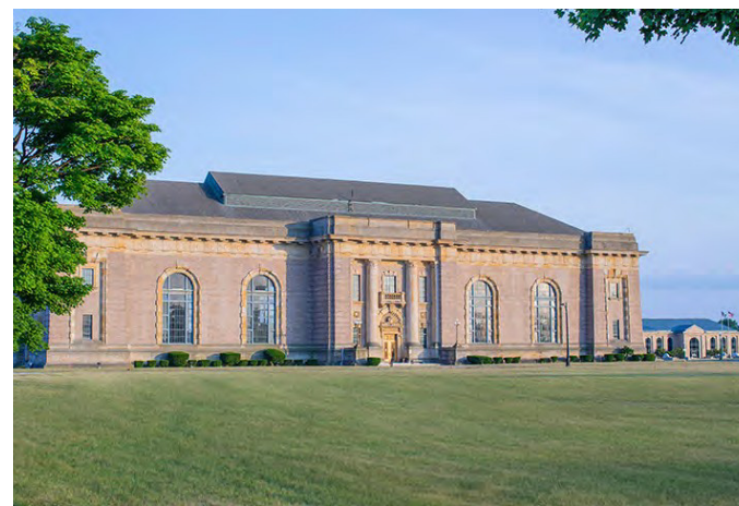
Figure 10. Water Works Park WTP
