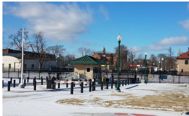
WWP security entrance from plant
