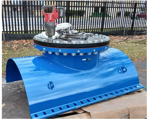
48-inch linestop sleeve ready for installation
