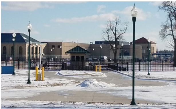
WWP security entrance from Jefferson Ave.
