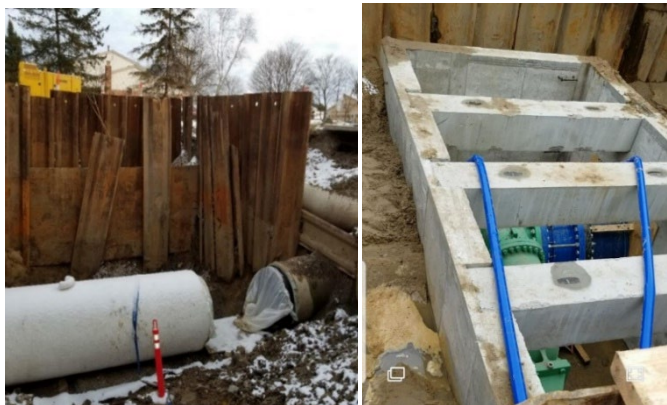
Before and after pictures of a gate valve installation
