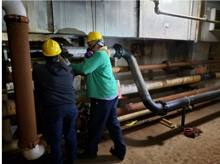
Dewatering team members installing new secondary water piping
