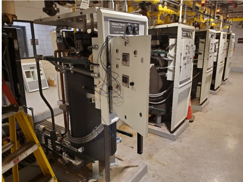
New Chlorine Evaporators (Trains #5 and #6) being Installed
