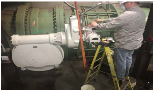
New conduit and electrical wiring installed for Valve V-12 Actuator
