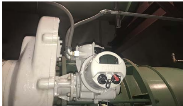
Valve V-12 completed conduit and electrical wiring
