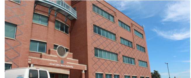
WRRF Facility Optimization Program
