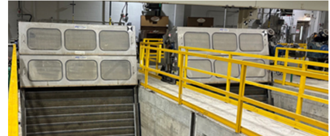
CSO Baby Creek Screen Rehabilitation
