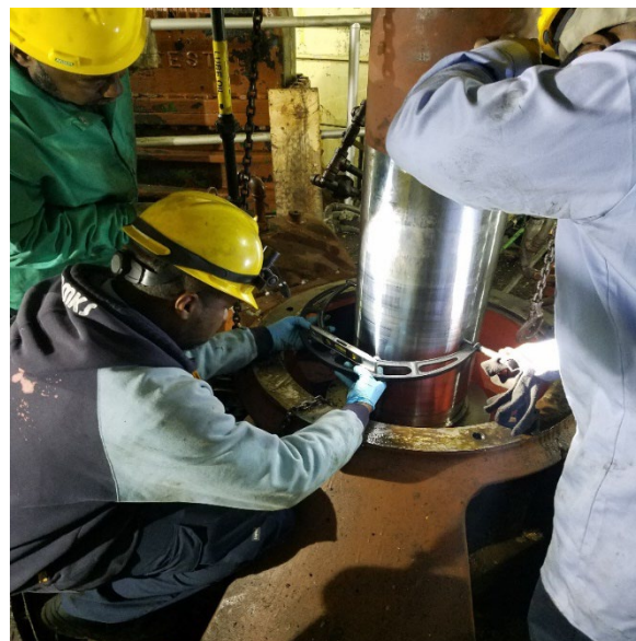
Primary Team Members measuring a shaft diameter
