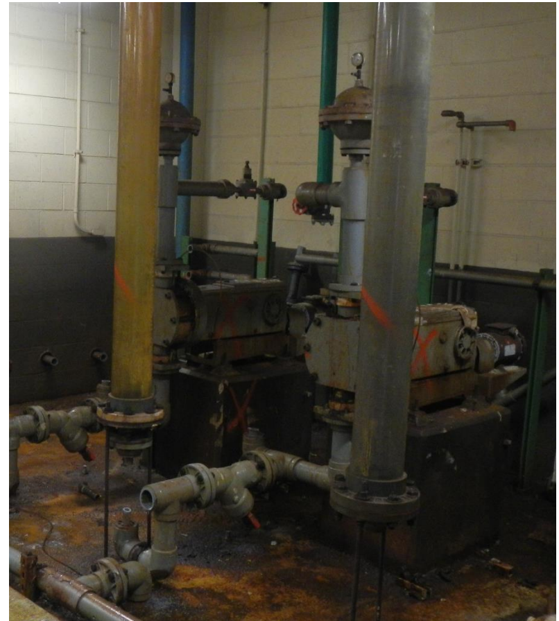
Demo of Existing Ferric Pumps/Piping
