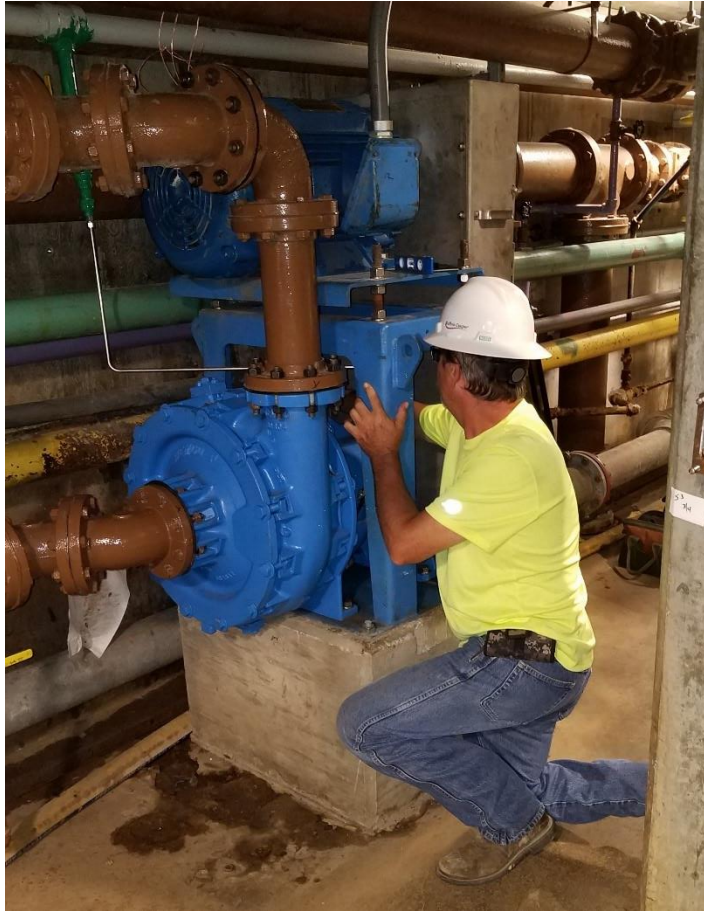
New Sludge Pump in Pipe Gallery
