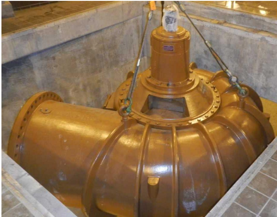
Lowering New Pump into Position
