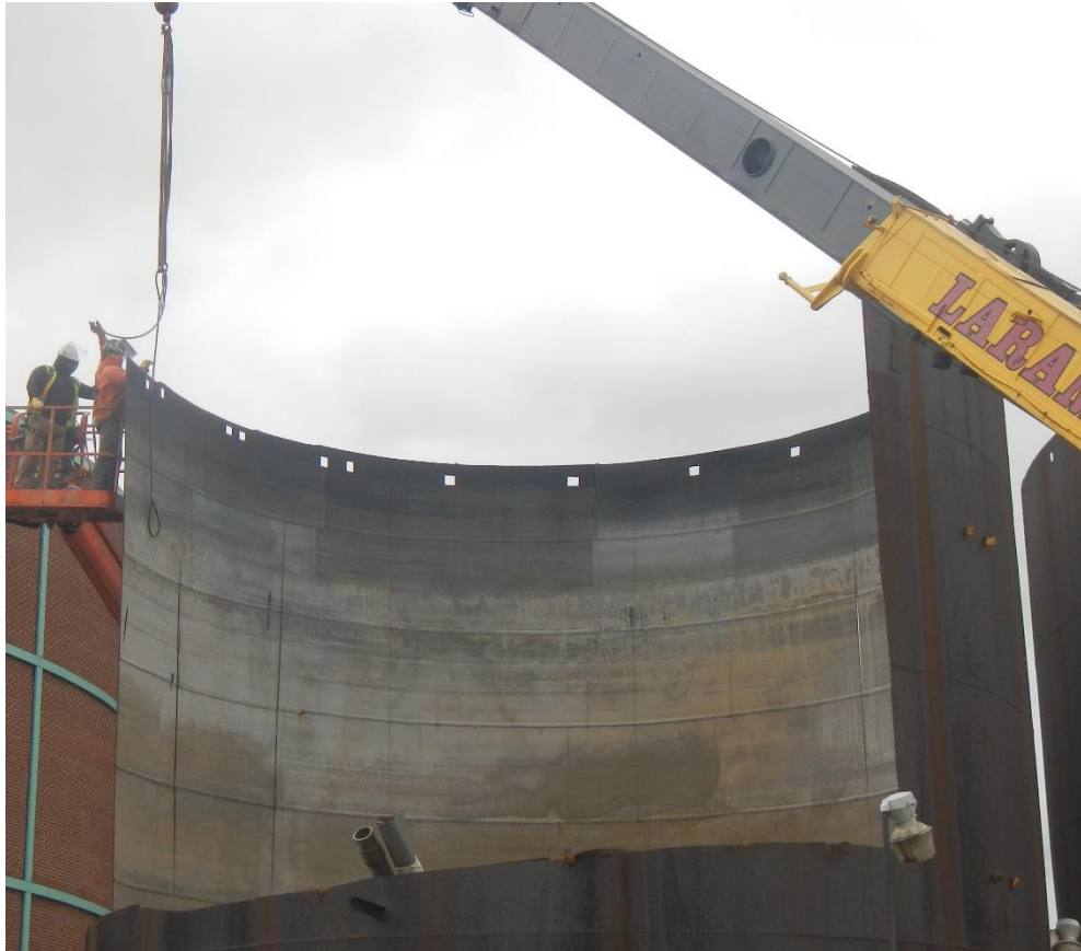
Demo of Existing Ferric Tanks
