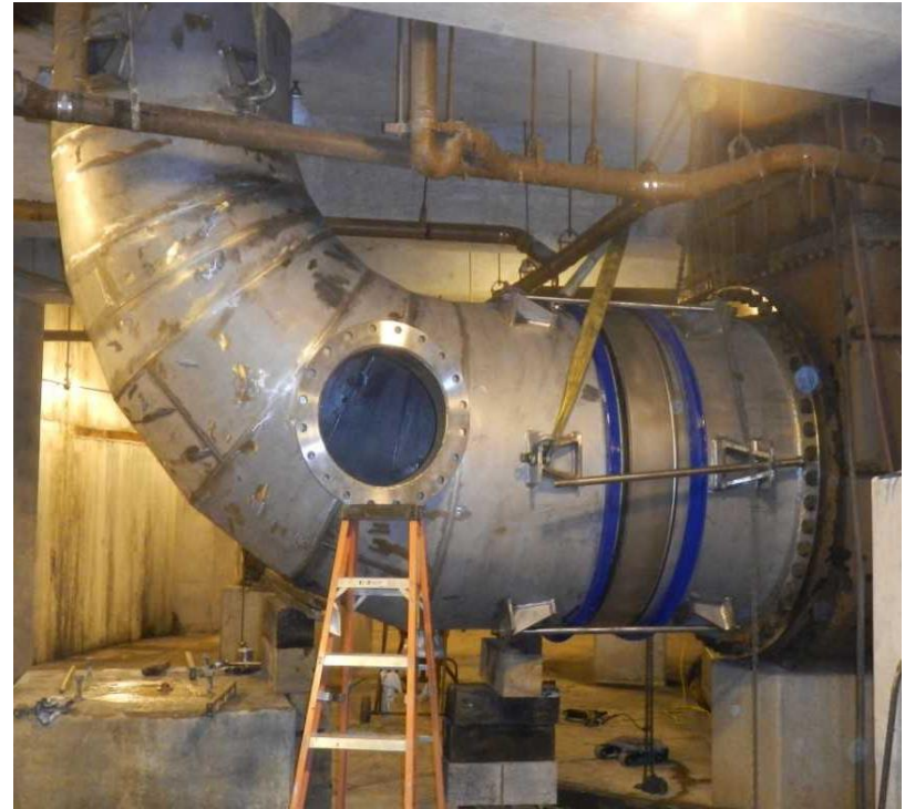
Suction Elbow Installation
