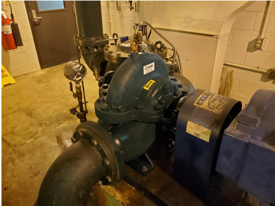
Refurbished booster pump
