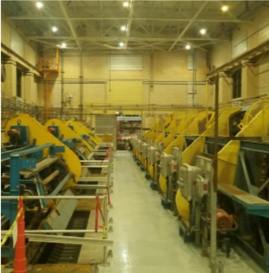
Bar Screens and Grit Collectors #5-8
