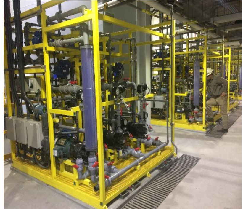
Chemical Feed Pump Skids
