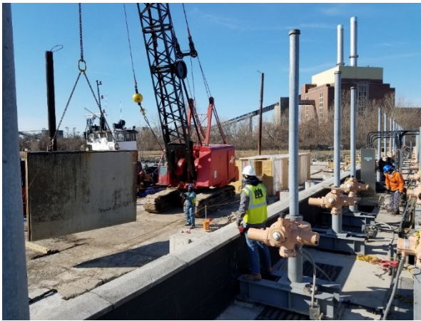
Replacing Seals on Effluent Relief Gates
