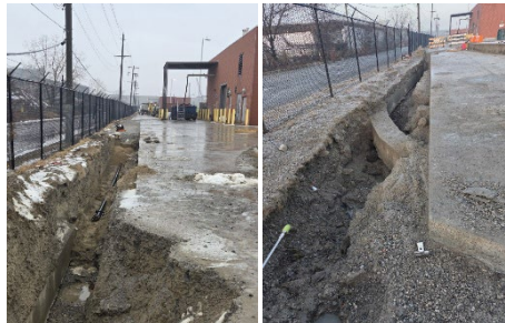
Scum line for PC 13 in the process of being replaced.
