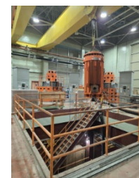
Sanitary Pump 10 at Freud SPS being lifted
