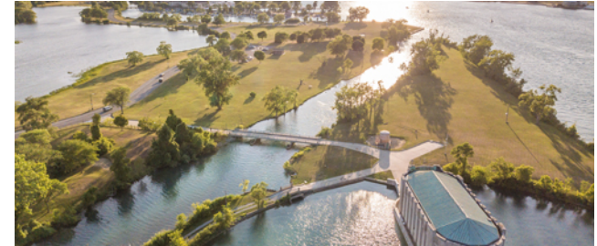
Belle Isle Intake System
