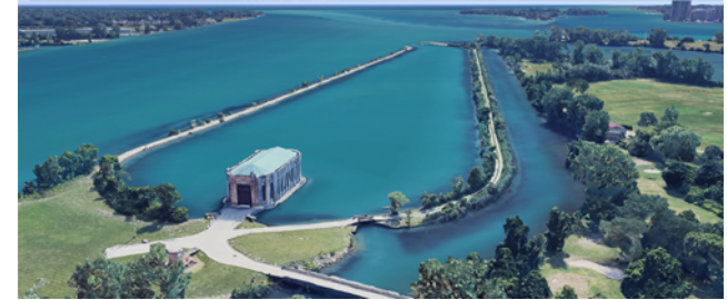
Belle Isle Seawall
