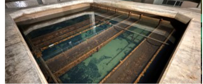
Northeast Water Treatment Plant Filter Replacement
