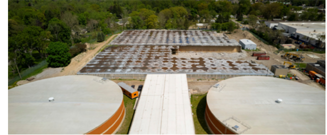
West Service Center Pumping Station
