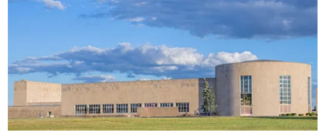
Northeast Water Treatment Plant
