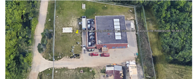
Ypsilanti Booster Pumping Station
