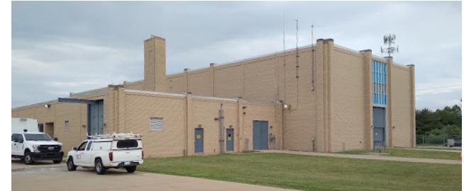
North Service Center Pumping Station
