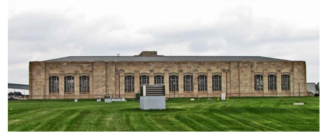
Springwells Water Treatment Plant
