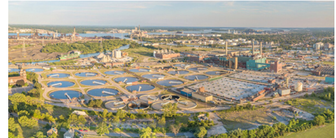
Low- and High lift Pumping station Improvements
