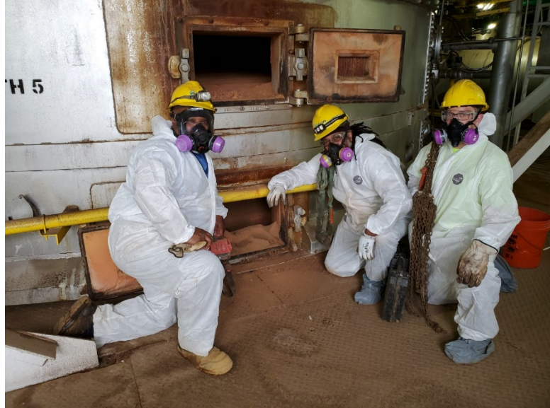
Incineration team members repairing Incinerator #11
