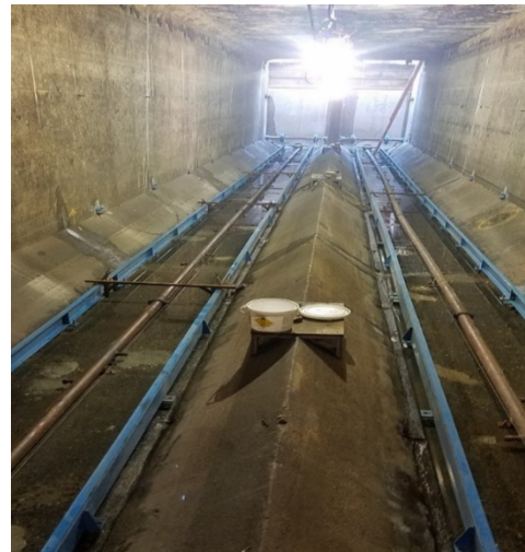
Underground grit channel prior to bucket installation
