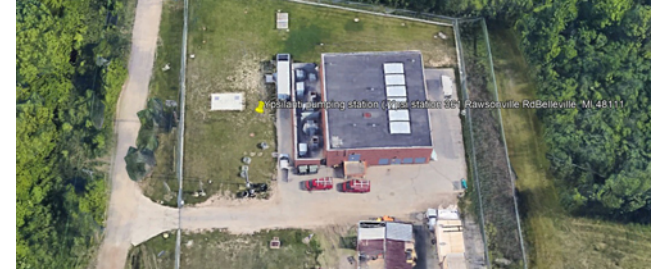
Ypsilanti Booster Pumping Station
