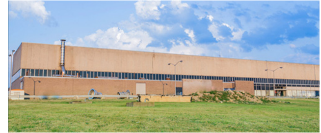
Southwest Water Treatment Plant
