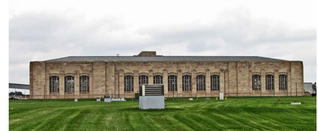
Springwells Water Treatment Plant
