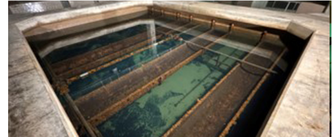
Northeast Water Treatment Plant Filter Replacement
