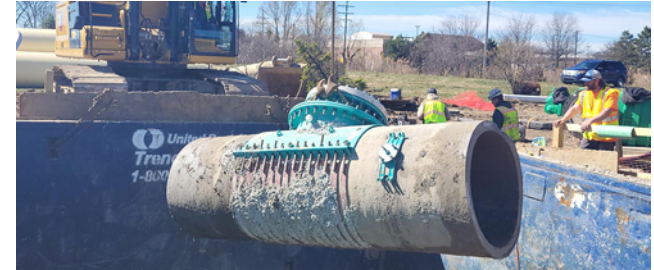
Transmission Mains Valves
