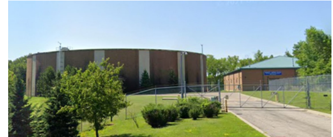
Imlay Pumping Station
