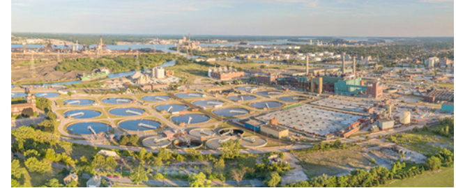
Low- and High lift Pumping station Improvements
