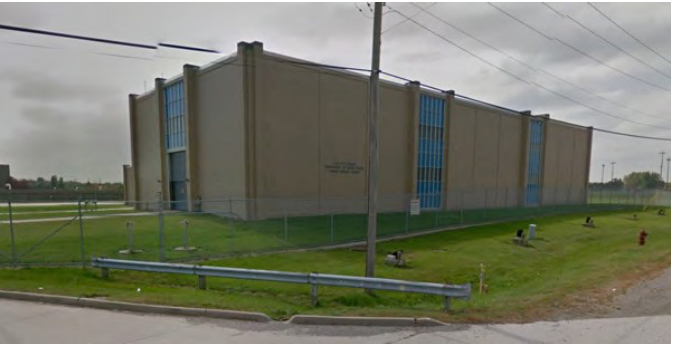
Figure 31. North Service Center
