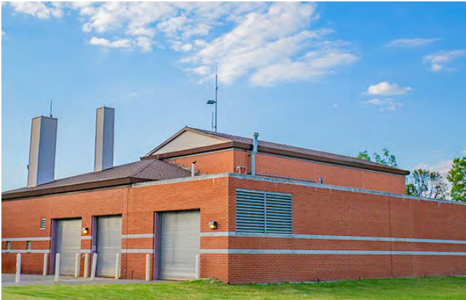
Figure 43. Puritan-Fenkell CSO RTB
