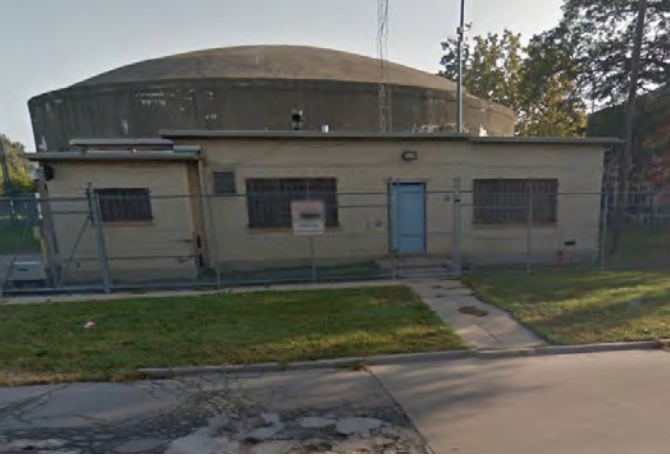
Figure 22. Electric Avenue Pump Station
