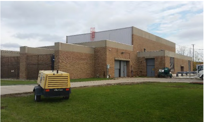
Figure 61. Northeast Pump Station
