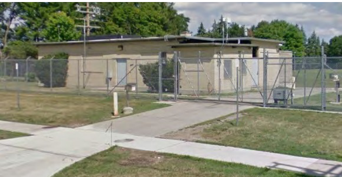
Figure 36. West Chicago Pump Station
