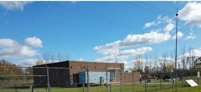
Figure 38. Ypsilanti Pump Station
