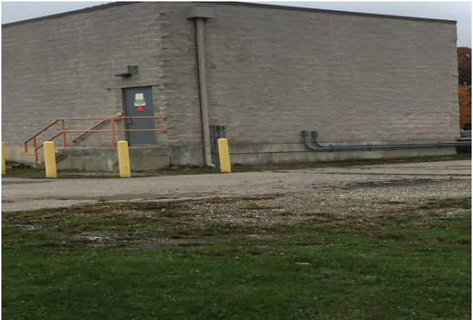
Figure 20. Adams Road Pump Station
