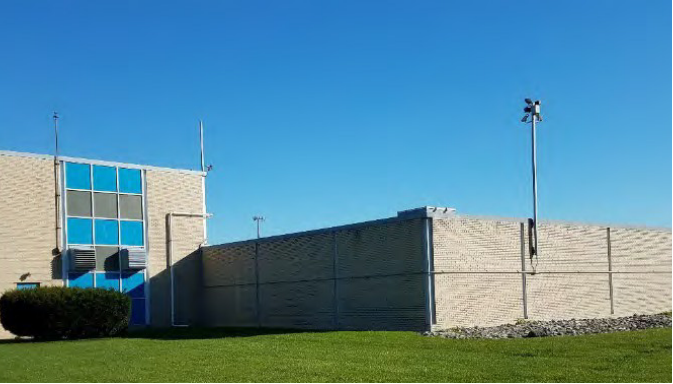
Figure 24: Ford Road Pump Station
