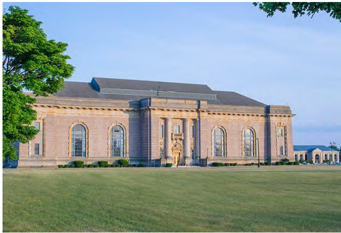
Figure 10. Water Works Park WTP
