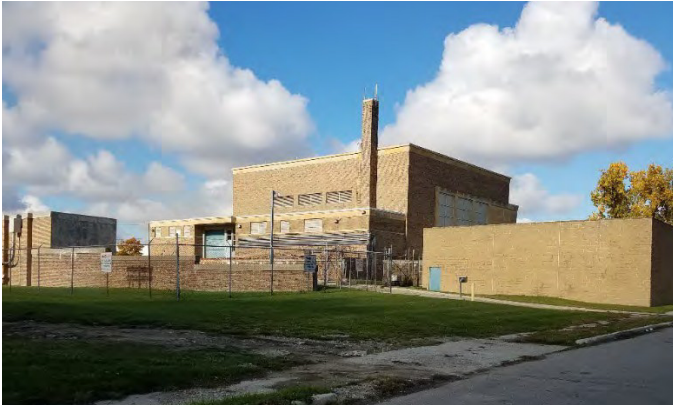
Figure 59. Freud Pump Station
