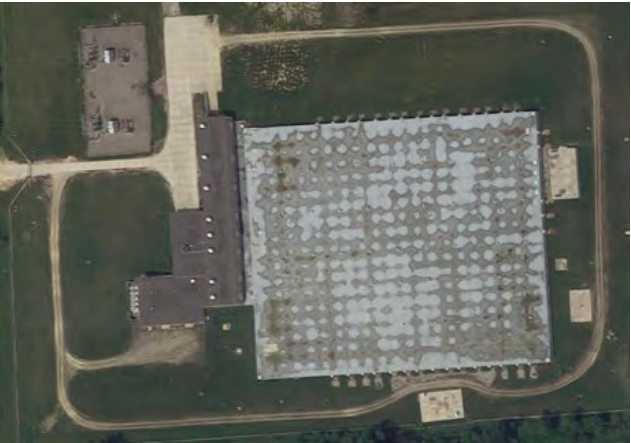
Figure 28. Imlay Pump Station
