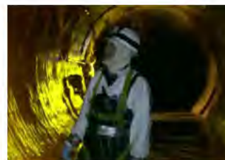
Visual inspection of a large sewer
