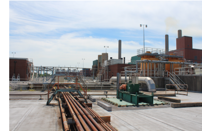
Aeration Basin 1 and ILP's 1 and 2
