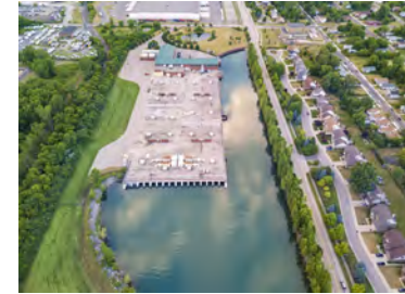
Conner Creek CSO Facility
