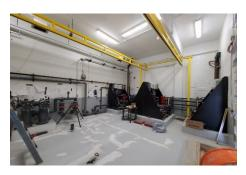
main work left for Package A is for ML-1 and PEAS-1 sampling stations. The main work left for Package B is electrical and controls work. Package A work is about 75% complete, and Package B is about 80% complete. The photo shows four Feed Pump Skids and a Dual Strainer installed in the FeCl Room.
