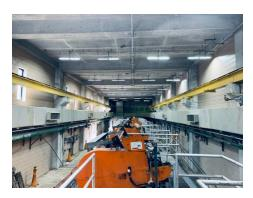
This project greatly improves visibility in the screenings building for our night-shift Plant Technicians while they are taking rounds or performing other required responsibilities. The photo shows the new LED lighting installed in the Pump Station 2 screenings area.
