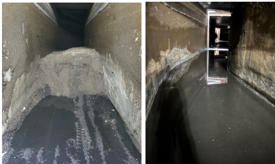
Before and after images of the cleaning effort in the PS-2 northside pump discharge channel
