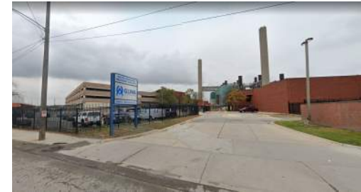
WRRF Front Entrance
