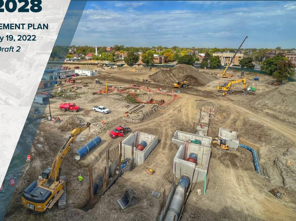
Water Works Park Water Treatment Plant Yard Piping, Valves, and Venturi Meters Replacement
