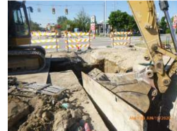
Construction on Merriman Rd.
