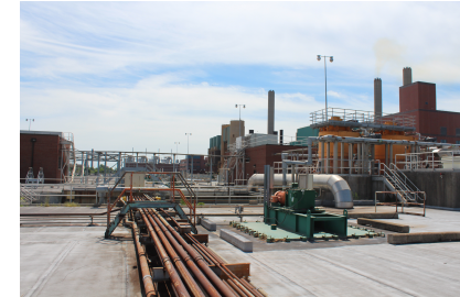
Aeration Basin 1 and ILP's 1 and 2
