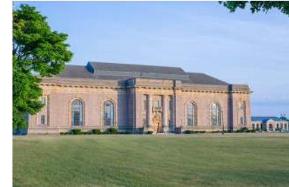
Water Works Park High Lift Pumping Station
