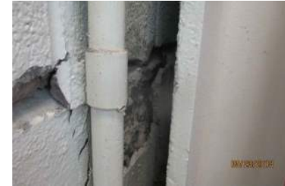
Existing Structural Condition
