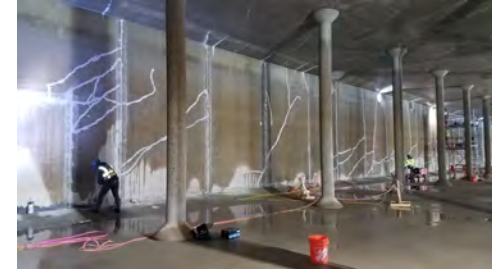
Imlay Booster Station: Sealing interior wall cracks
