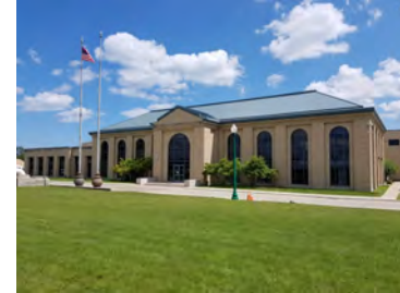
Water Works Park Water Treatment Plant
