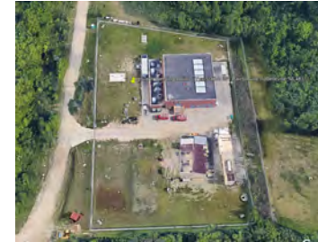
Existing Ypsi station
