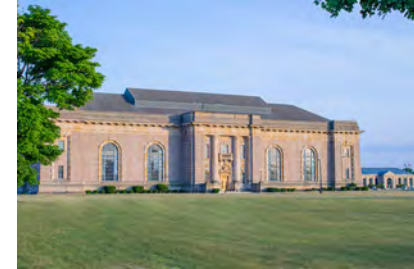
Water Works Park High Lift Pumping Station
