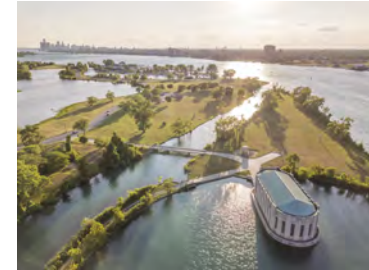
Belle Isle Intake
