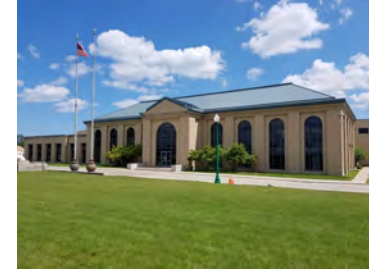
Water Works Park Water Treatment Plant
