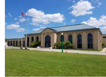
Photo of Water Works Park Plant
