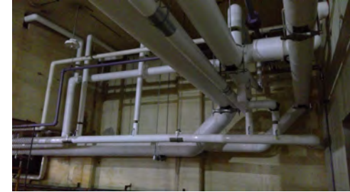
Maintenance building photo 1 of finished section of piping
