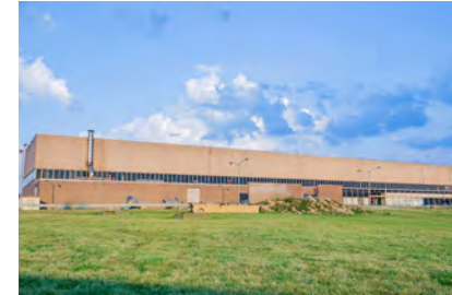
SW SCADA System Upgrade
