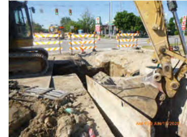
Construction on Merriman Rd.
