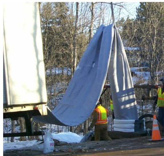
Figure 3 - Example of cured-in-place pipe installation
