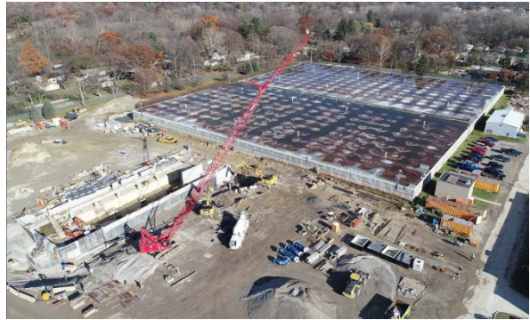
Aerial Project Overview
