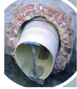
Figure 2 - Sliplining Non-Circular Pipe
