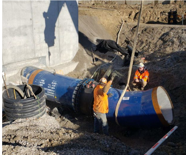
Installation of 42" reservoir outlet piping
