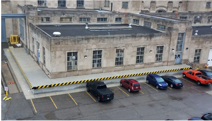
New loading dock
