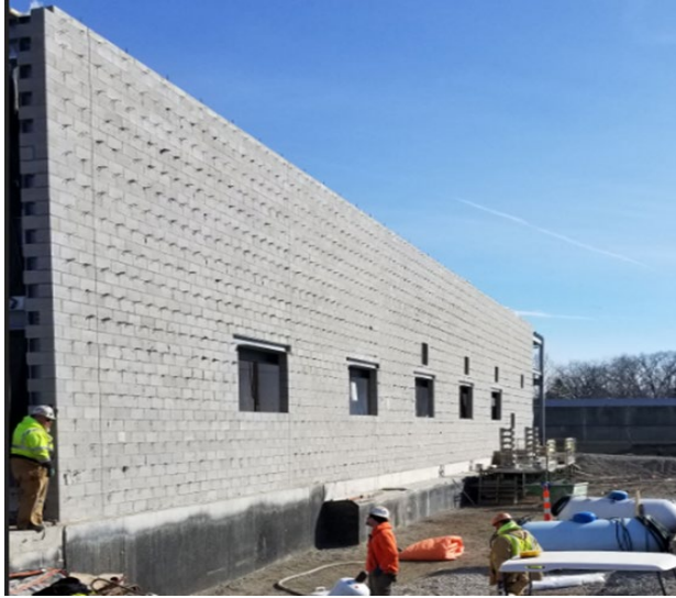
New reservoir pump house masonry wall in progress
