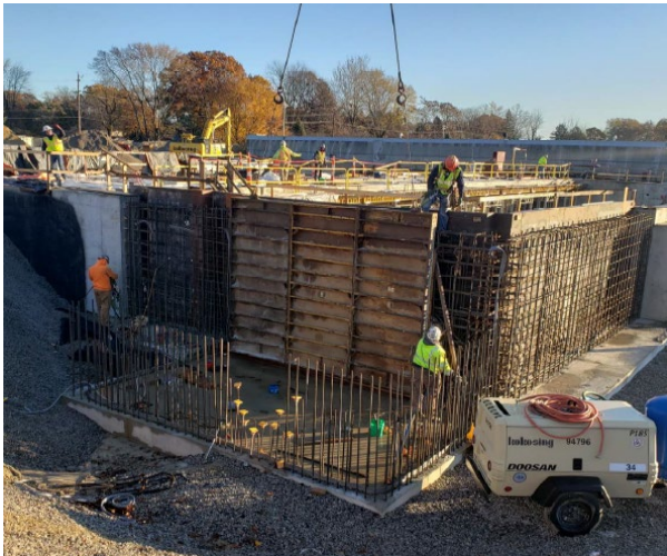
New reservoir pump house wall formwork and reinforcing
