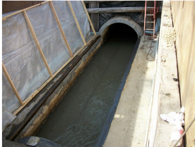
Figure 4 - Pipe opened up for sliplining at insertion pit
