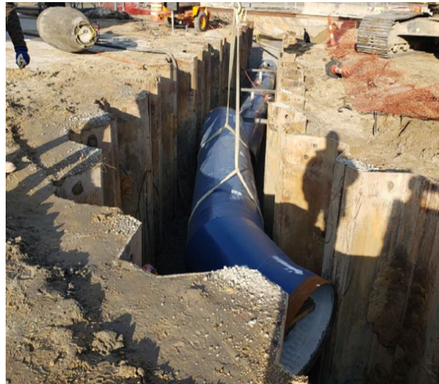
Installation of 42" reservoir pump house discharge piping
