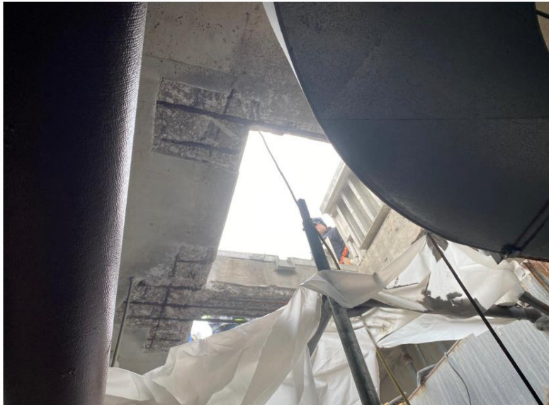
Photo 3: Pullman and Wade Trim looking at deteriorated expansion joint.
