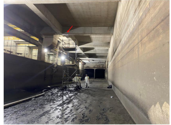
Photo 2: The arrow indicates the structural injection on the underside of the beam.
