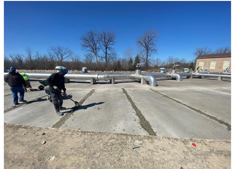
Photo 4: Pullman distributing concrete into open joints.
