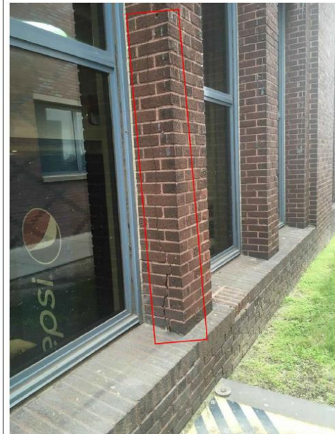
PHOTO 3 — TYPICAL BROKEN BRICK OLD ADMINISTRATION BUILDING
