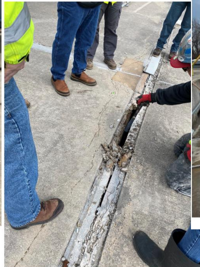
Photo 3: Pullman and Wade Trim looking at deteriorated expansion joint.
