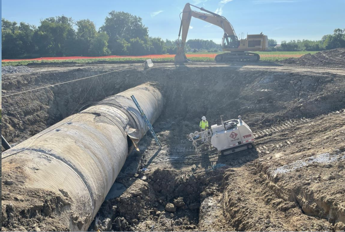
Removal of Damaged Pipe
