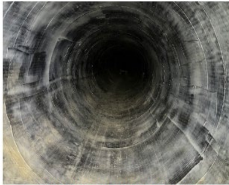
Looking E at pipe 213 to completed CFRP lining
