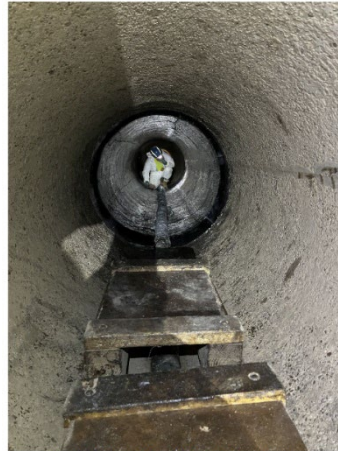
Looking E at Pipe 262 installed layers
