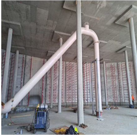
Reservoir 2 reservoir filled 24-inch pipe installation
