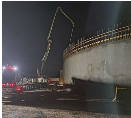
Reservoir 1 roof deck concrete placement east half
