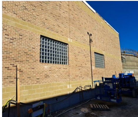
Pump station glass block window installation
