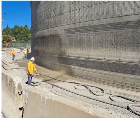
Reservoir 2 shotcrete wire cover and cover
