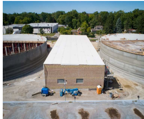
Aerial view of new pump house
