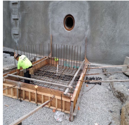
Reservoir 1 overflow structure foundation slab formwork and reinforcing steel installation
