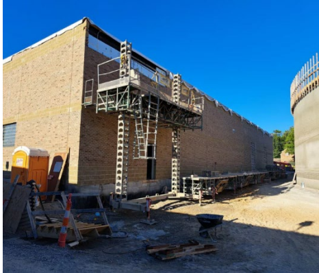
Pump station masonry face brick installation (north side of building)
