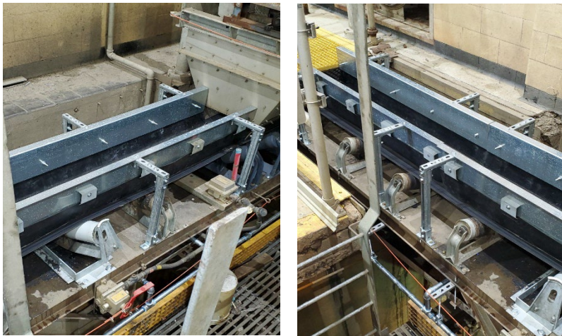
The addition of skirting to the skybelt will reduce the amount of grit falling off the belt improving the overall cleanliness of PSI Rack and Grit
