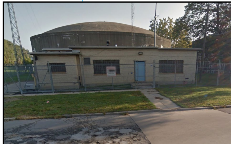
Figure 22. Electric Avenue Pump Station
