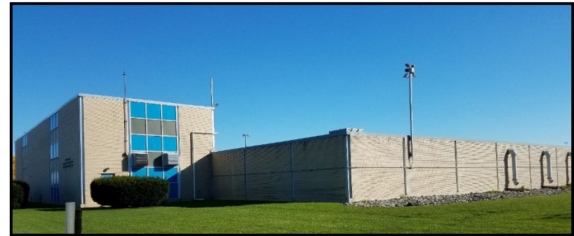
Figure 24. Ford Road Pump Station
