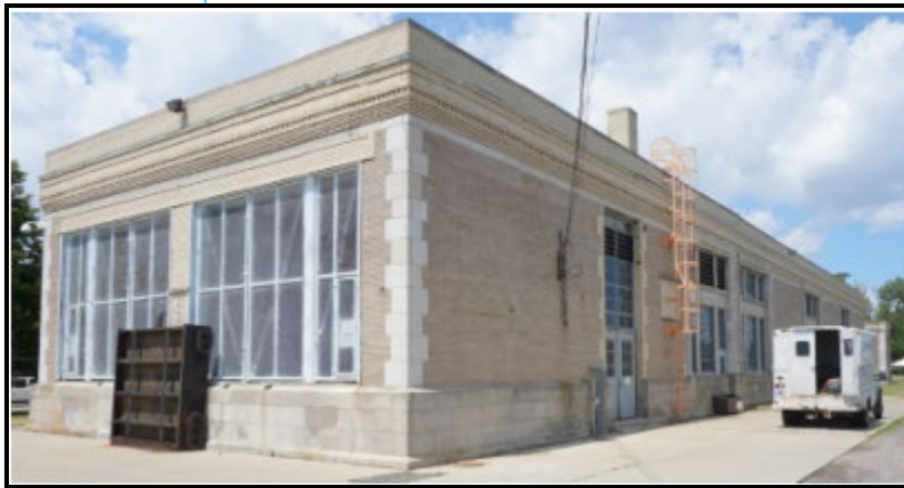
Figure 57. Fairview Pump Station
