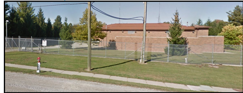
Figure 33. Rochester Pump Station
