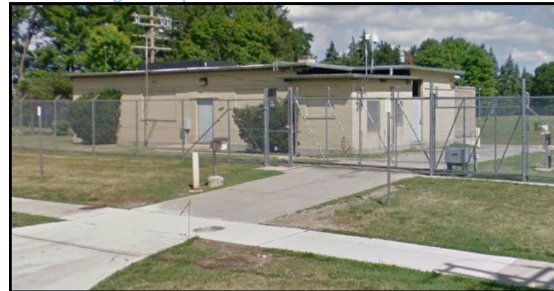
Figure 36. West Chicago Pump Station
