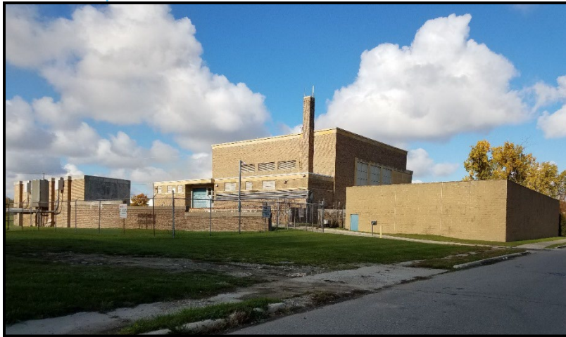
Figure 59. Freud Pump Station
