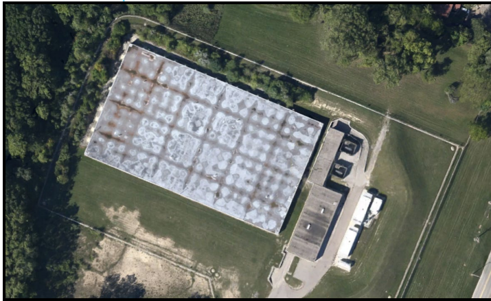
Figure 25. Franklin Pump Station
