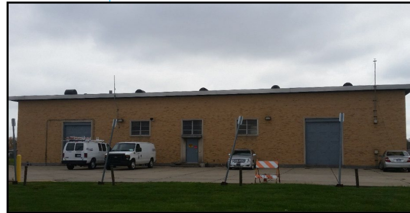
Figure 30. Northwest Pump Station
