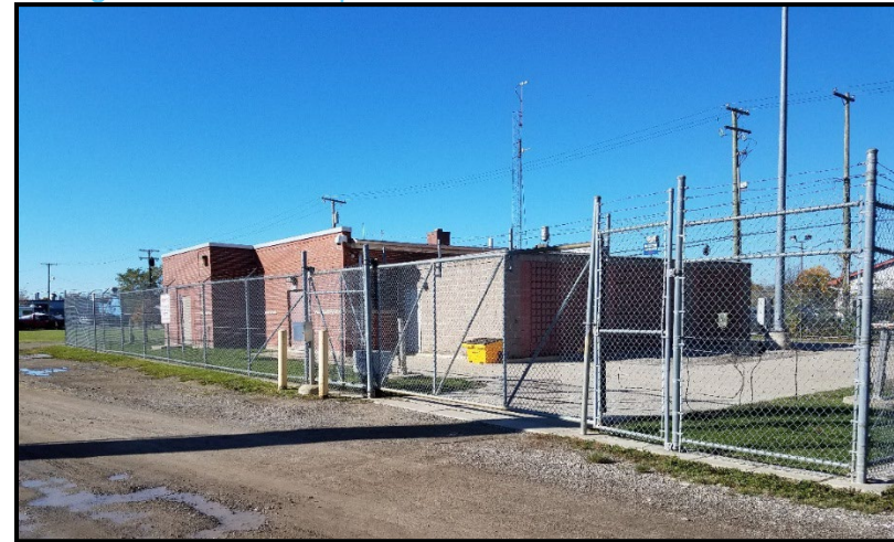
Figure 26. Michigan Avenue Pump Station
