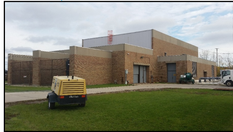
Figure 61. Northeast Pump Station
