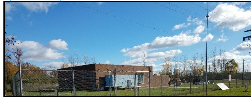
Figure 38. Ypsilanti Pump Station
