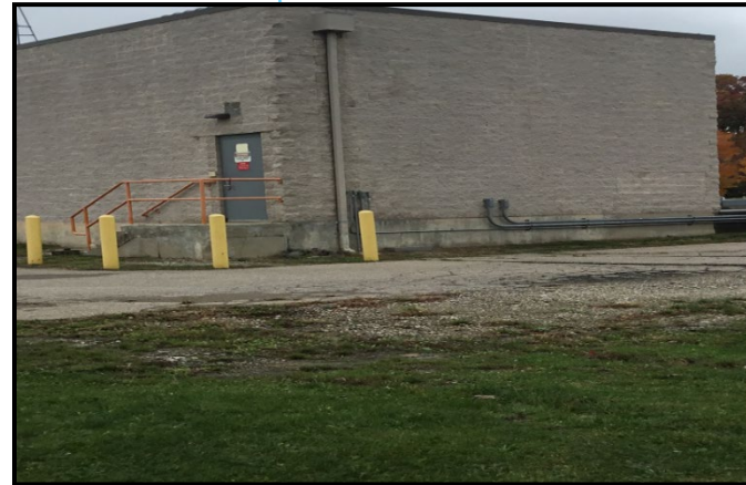
Figure 20. Adams Road Pump Station
