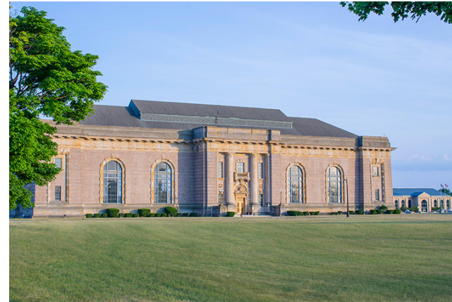
Figure 10. Water Works Park WTP
