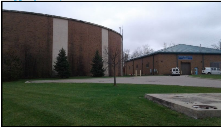
Figure 23. Haggerty Pump Station
