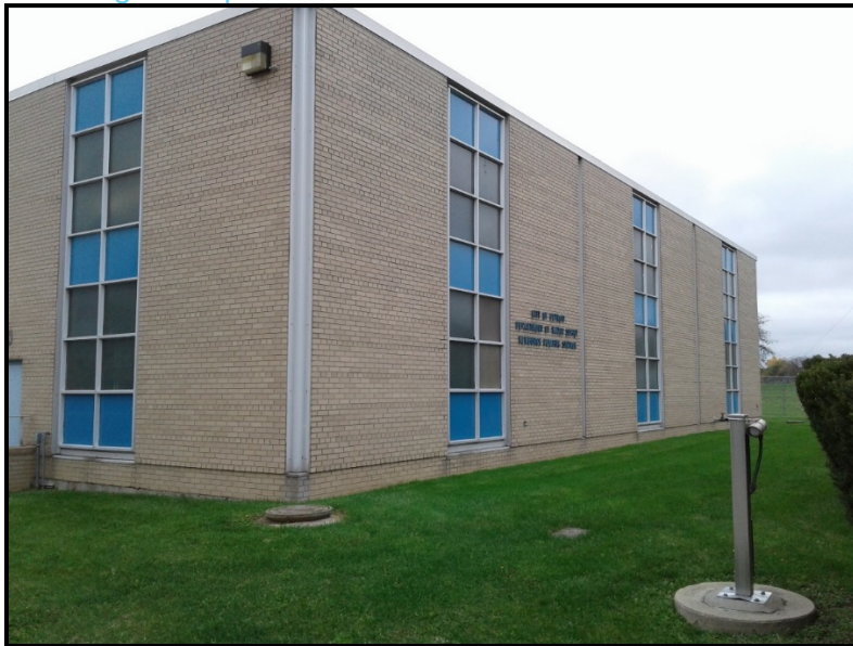
Figure 29. Newburgh Pump Station
