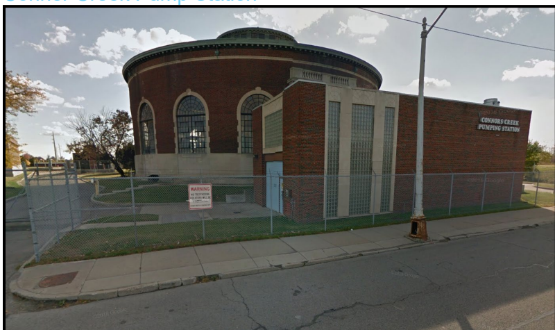
Figure 55. Conner Creek Pump Station
