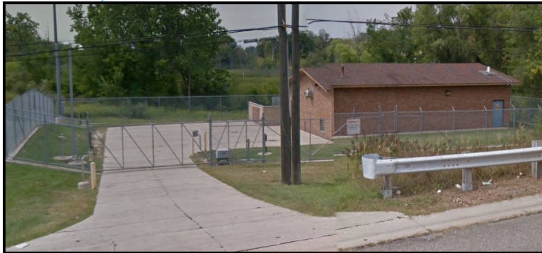
Figure 32. Orion Pump Station
