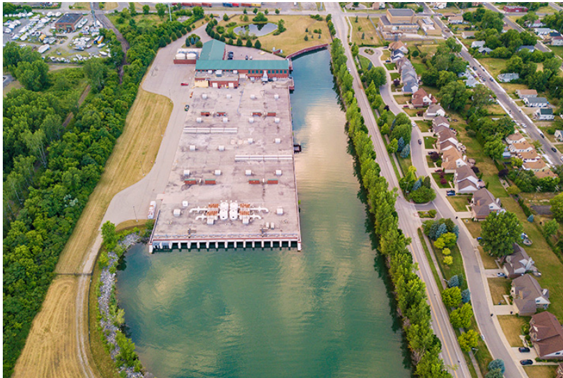
Figure 40. Conner Creek CSO RTB
