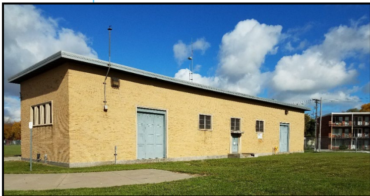
Figure 21. Eastside Pump Station
