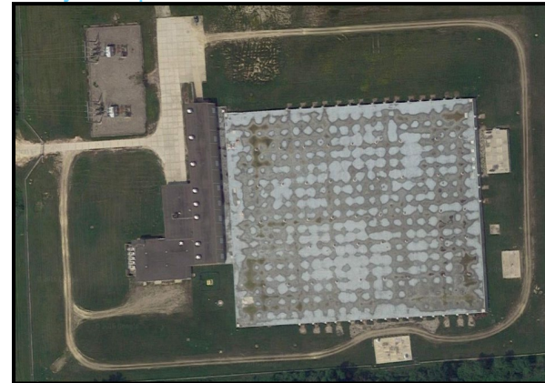
Figure 28. Imlay Pump Station
