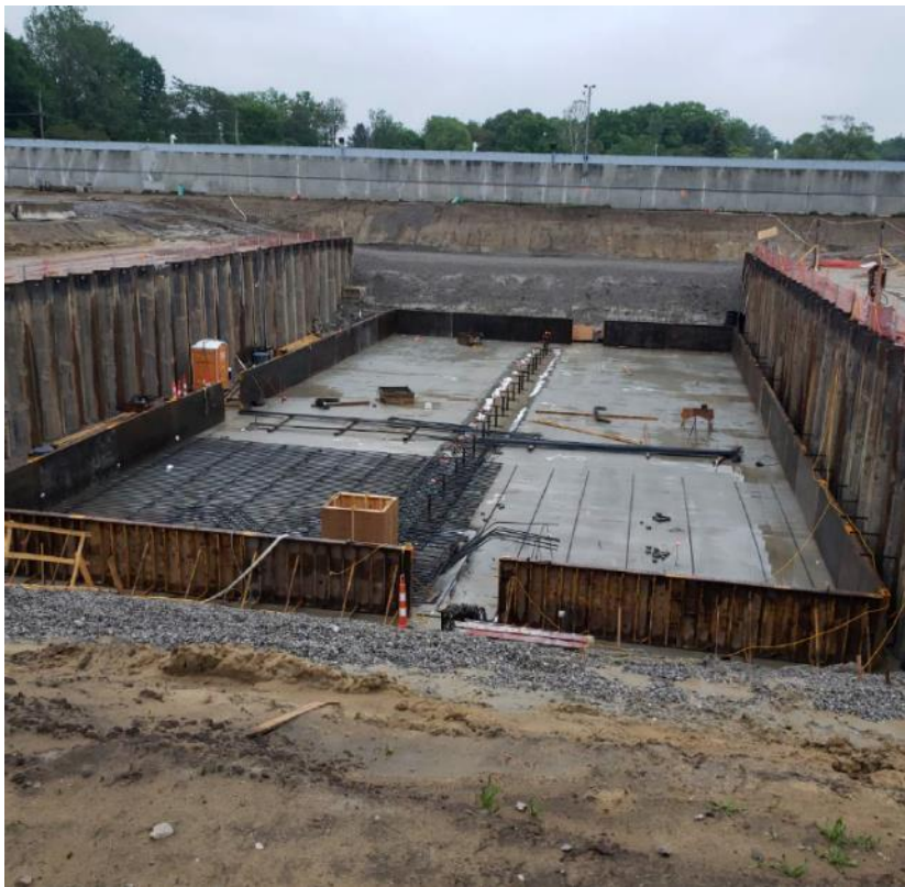
New Reservoir Pump House Base Slab Progress
