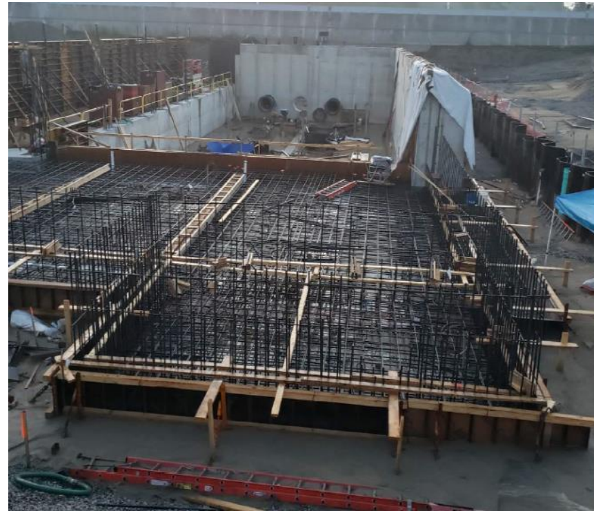
New Reservoir Pump House – Fill Valve Slab Forms and Reinforcement
