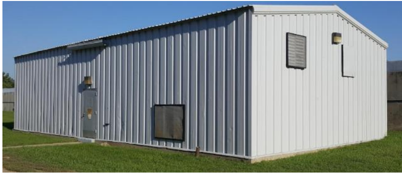
Existing Reservoir Pump Houses No. 1 and No. 2
