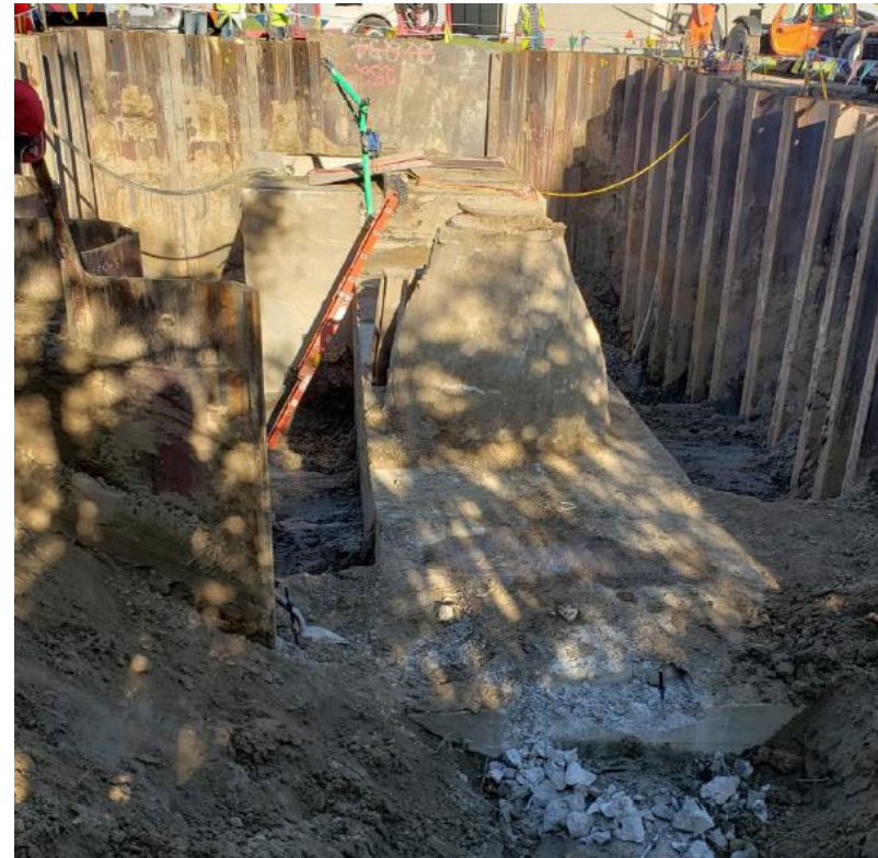
Valve Well No. 3 Excavation Complete
