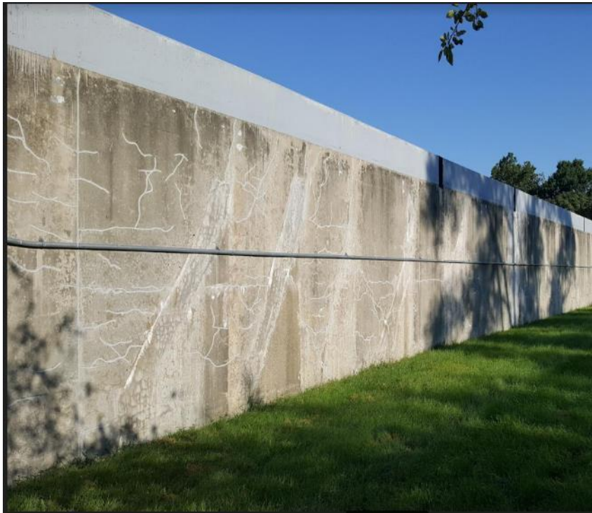
Existing Reservoir No. 1 East Exterior Wall
