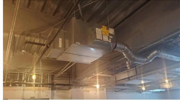
*Fan Powered Variable Air Volume (VAV) installation in progress*
