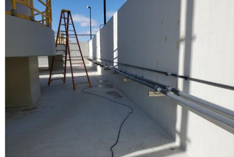
*Damaged Ferric Chloride discharge piping is replaced by the Contractor shown above*
