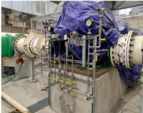
*Horizontal Split Case (HSC) pump impulse piping Instrumentation Rack*
