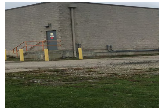
Figure 20. Adams Road Pump Station
