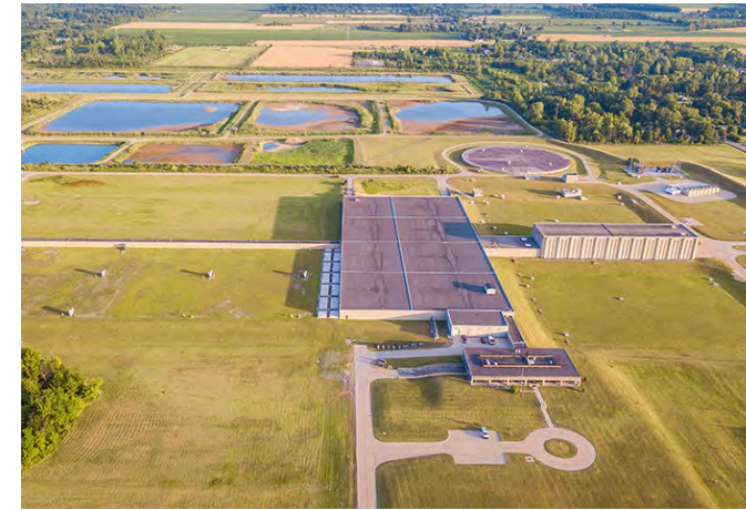
Figure 3. Lake Huron WTP
