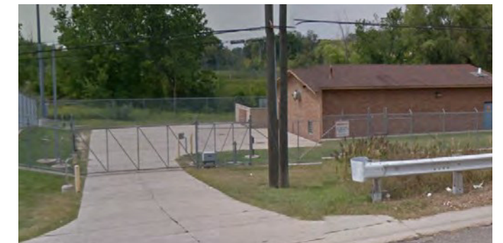
Figure 32. Orion Pump Station
