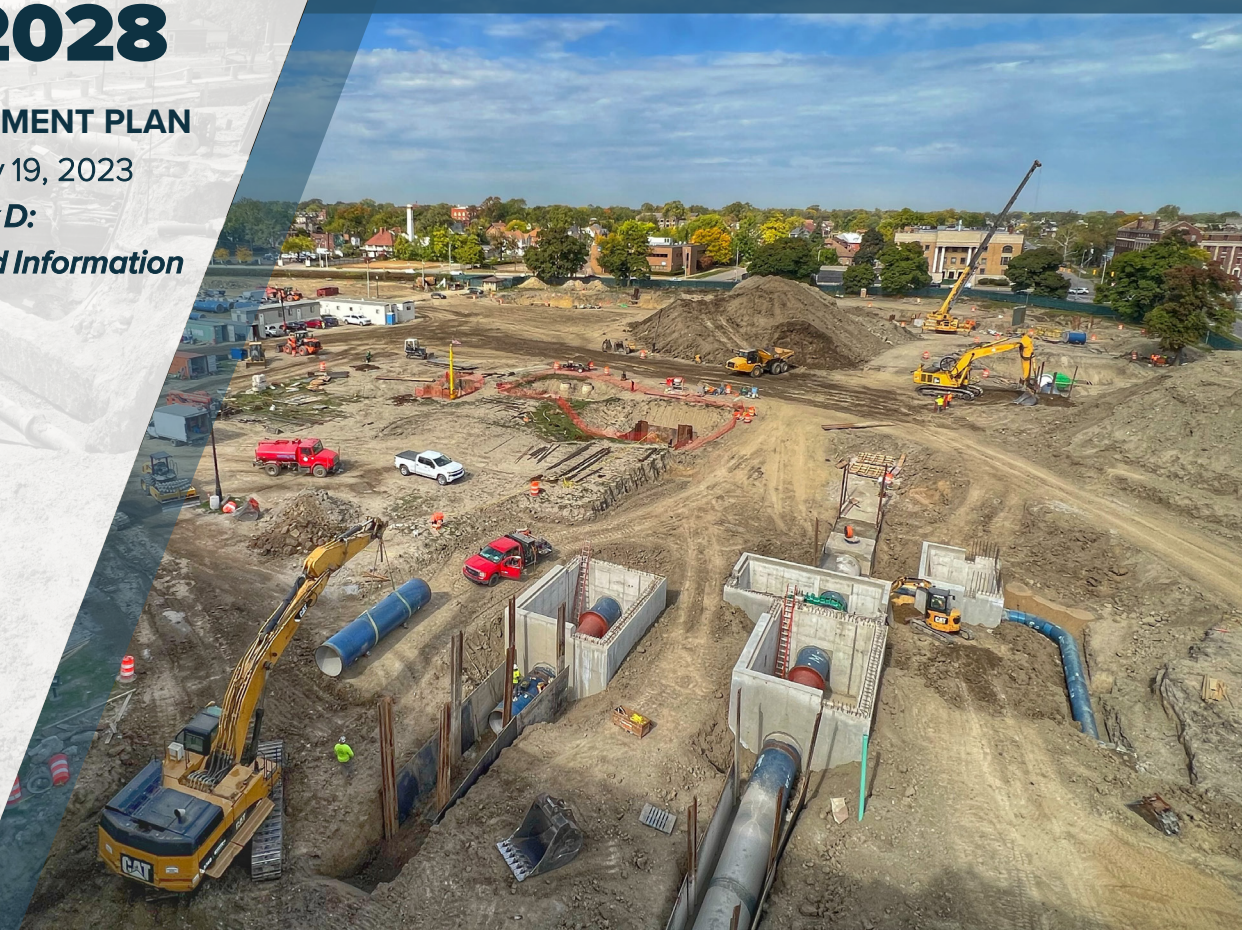
Water Works Park Water Treatment Plant Yard Piping, Valves, and Venturi Meters Replacement Photo submitted by: Jacob Magnum of Water and Field Services
