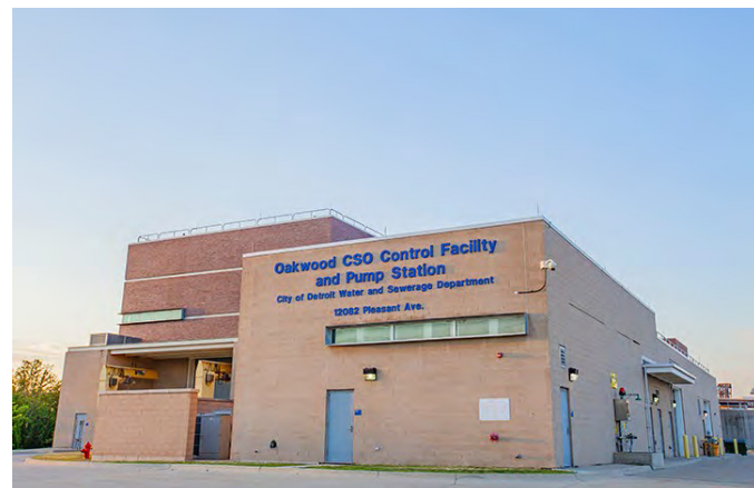
Figure 42. Oakwood CSO RTB
