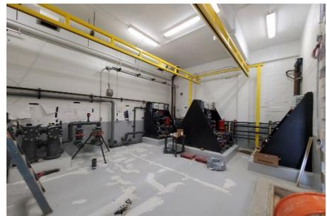
The PEAS-1 cost proposal is under review by GLWA. The main work left for Package A is for ML-1 and PEAS-1 sampling stations. The main work left for Package B is electrical and controls work. Package A work is about 75% complete, and Package B is about 80% complete. The photo shows four Feed Pump Skids and a Dual Strainer installed in the FeCl Room.
