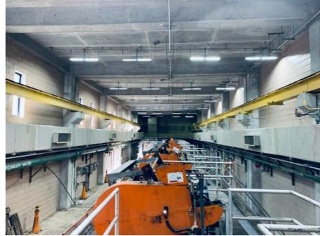
This project greatly improves visibility in the screenings building for our night-shift Plant Technicians while they are taking rounds or performing other required responsibilities. The photo shows the new LED lighting installed in the Pump Station 2 screenings area.
